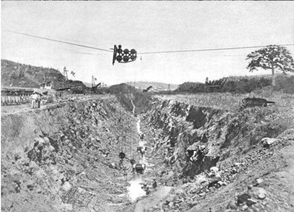
Top Left: caption: “View of the Canal at Emperor, on the Western Slope of the Divide. The American Cableway is in use removing materials from the trench”
