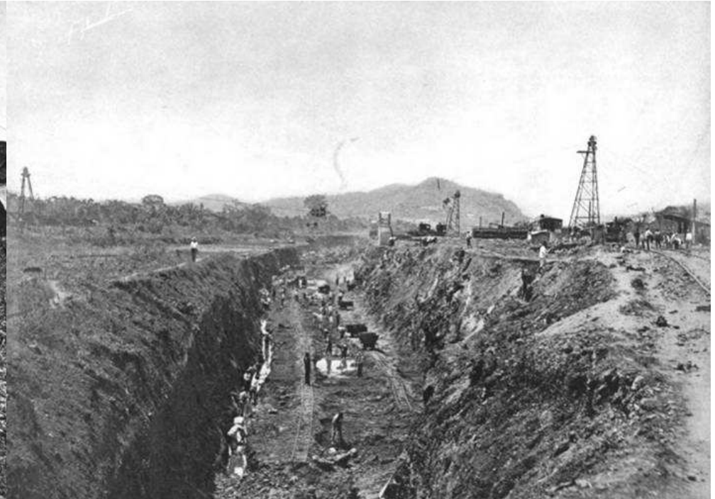
Top Left: caption: “View of the Canal at Emperor, on the Western Slope of the Divide. The American Cableway is in use removing materials from the trench”
