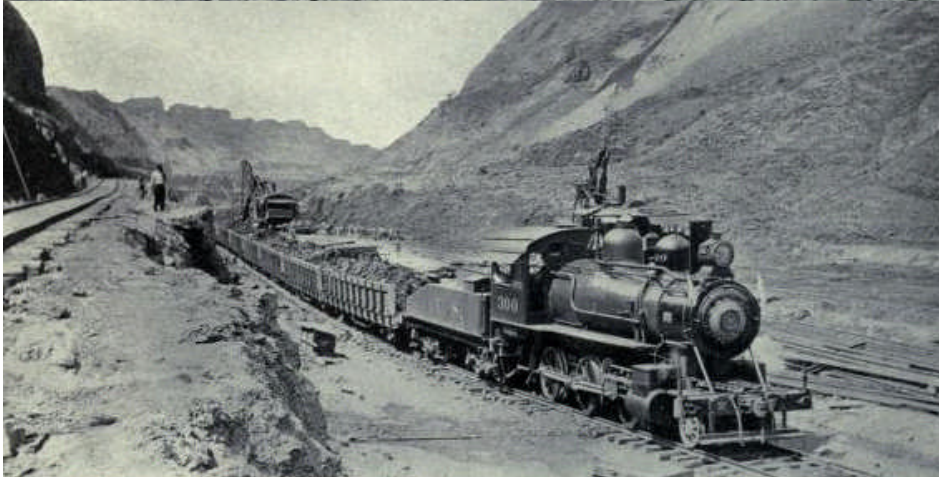
Top Left: caption: “As the shovels load a car, the locomotive pushes the train along slowly until the whole train is full. Then off to the dump and back for another load.”
