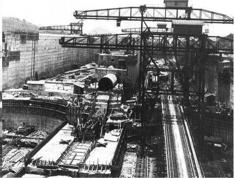
Top Left: caption: “Miraflores Upper Locks. Upper end of Center Wall, showing Gate Protection Castings and Cylindrical Valves, July 1911”
