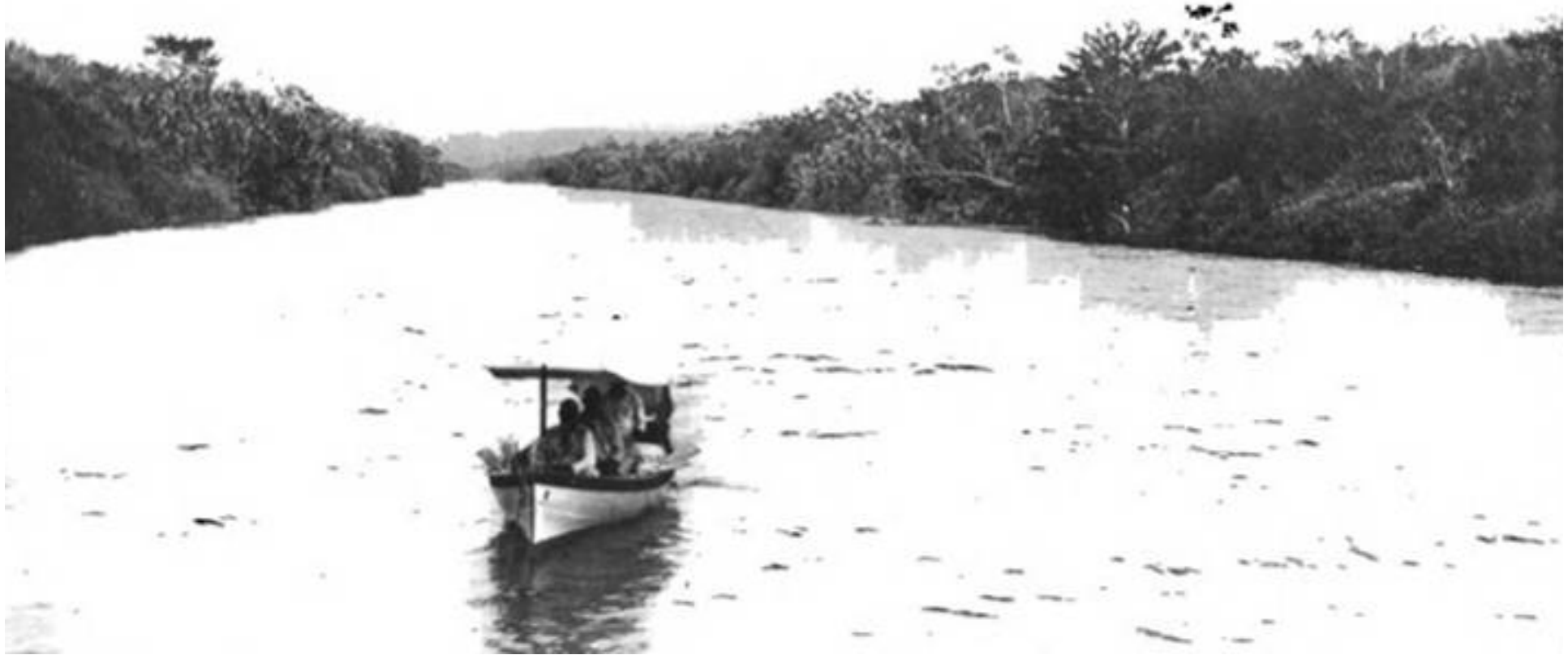
5.—COMPLETED CANAL, 10 MILES FROM ITS ATLANTIC ENTRANCE. CANAL IS EXCAVATED TO WIDTH SHOWN FOR 15 MILES, OR UP TO BOHIO.
