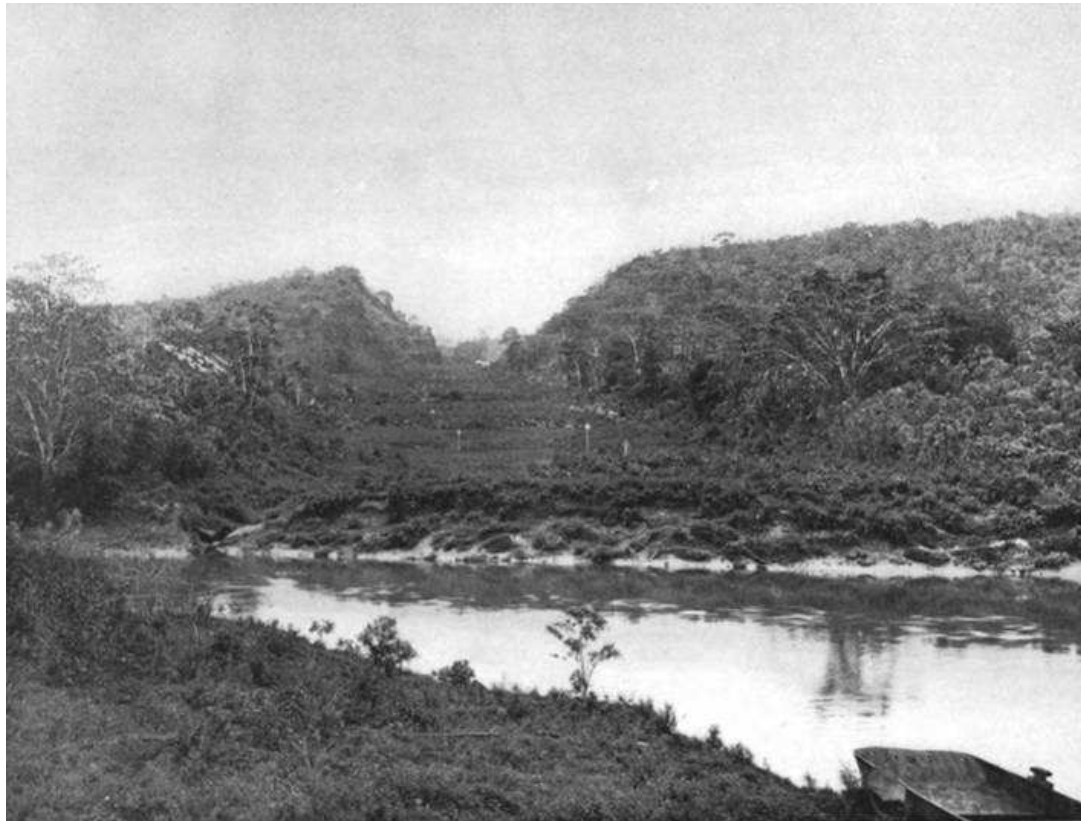
3 —BOHIO—SITE OF LOCKS AND DAM. CHAGRES RIVER IN THE FOREGROUND. LOCKS WILL BE BUILT IN THE DEEP CUT BEYOND THE RIVER.
