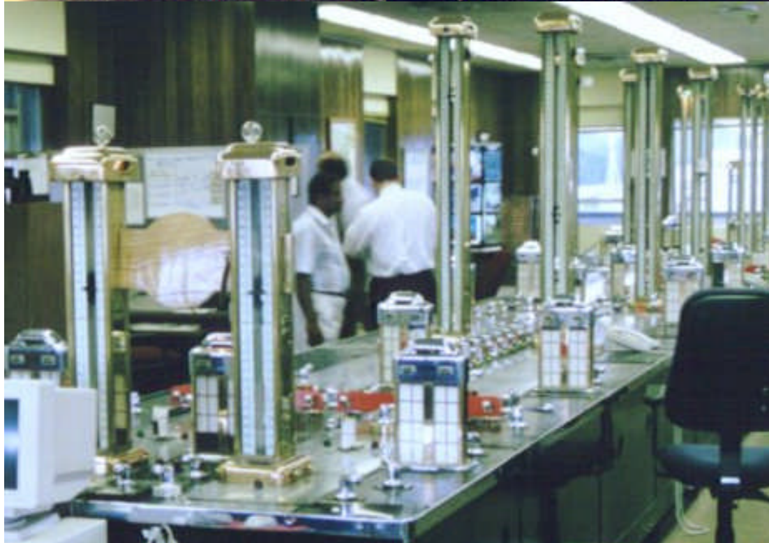
Control tower Interior ~ Panama Canal
