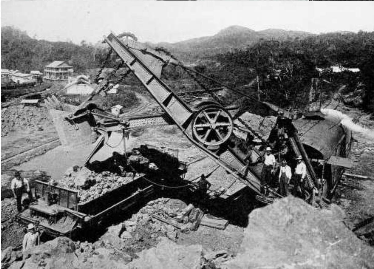
Top Left: caption: “A Marion steam shovel excavating the Panama Canal in 1908”
