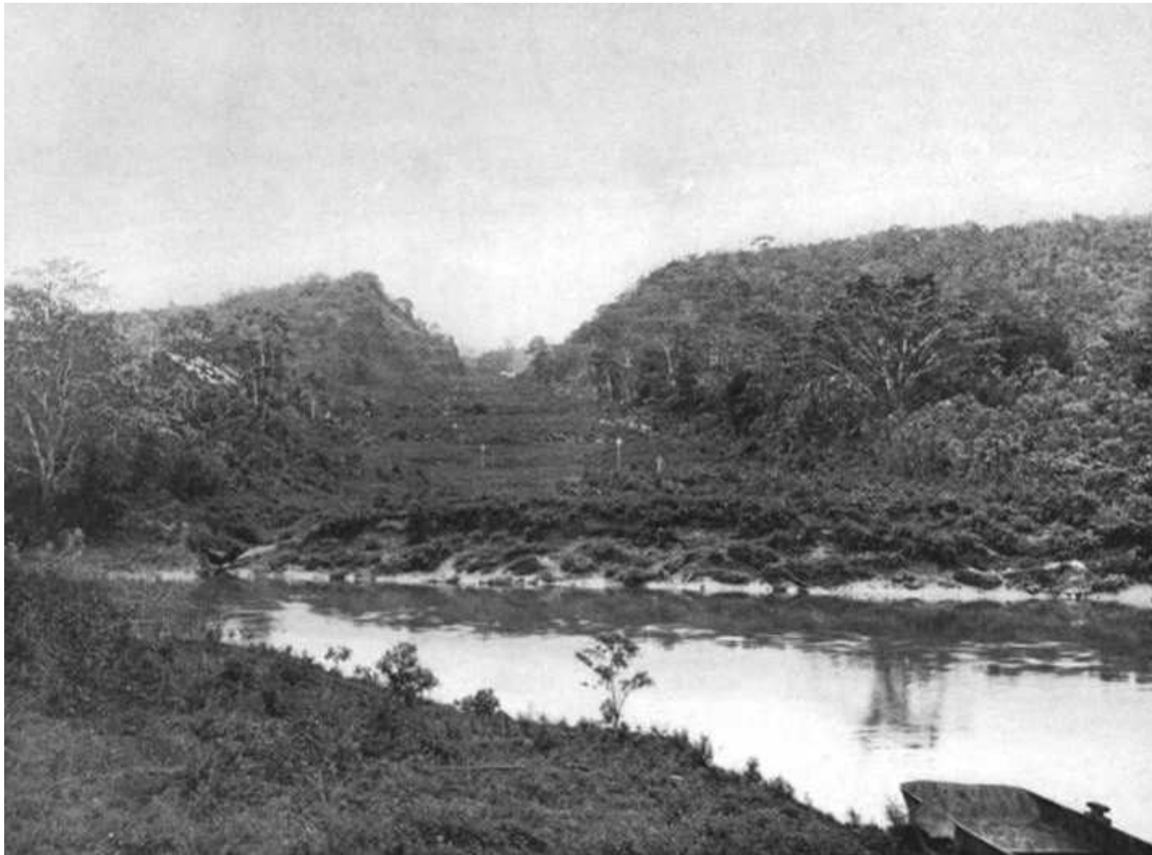
Above: caption: “View of the excavation at Bohio”
