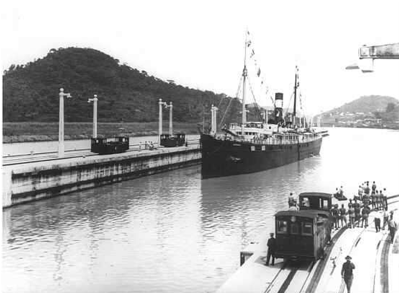
Above: caption: “SS Advance arriving at Pedro Miguel Locks, going south on trip through canal. Attaching lines from towing locomotives, August 1914”
