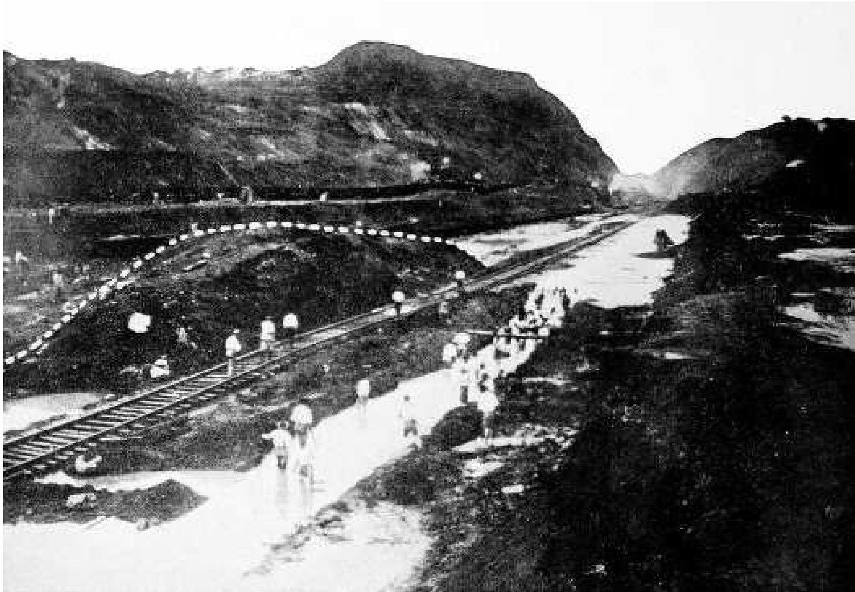
Above: caption: “An Eruption of the Canal Bed.’ The pressure of the adjoining hills has forced up the soil at its weakest point, namely the bed of the Canal, to a height of 18 feet, as shown by the dotted line.” 601
