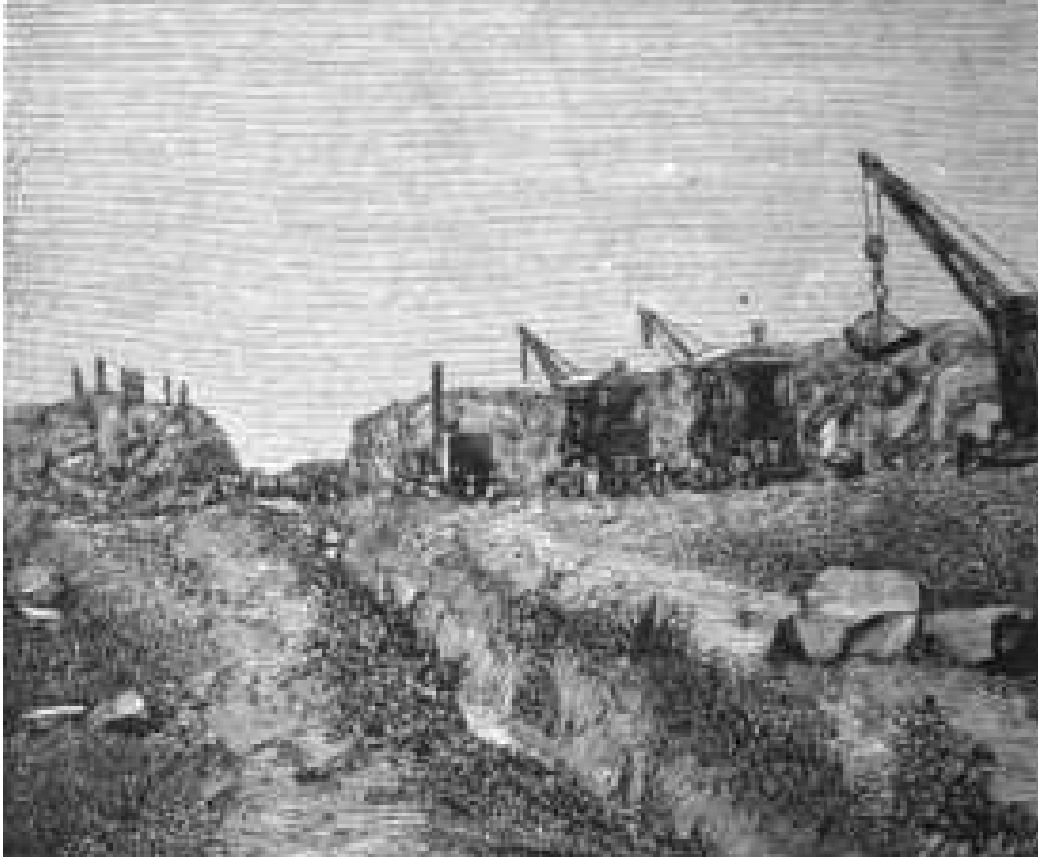
Top Left: caption: “A French excavator opening a pioneer trench in the south end of the Cut. This was the best known method of excavating in that day”
