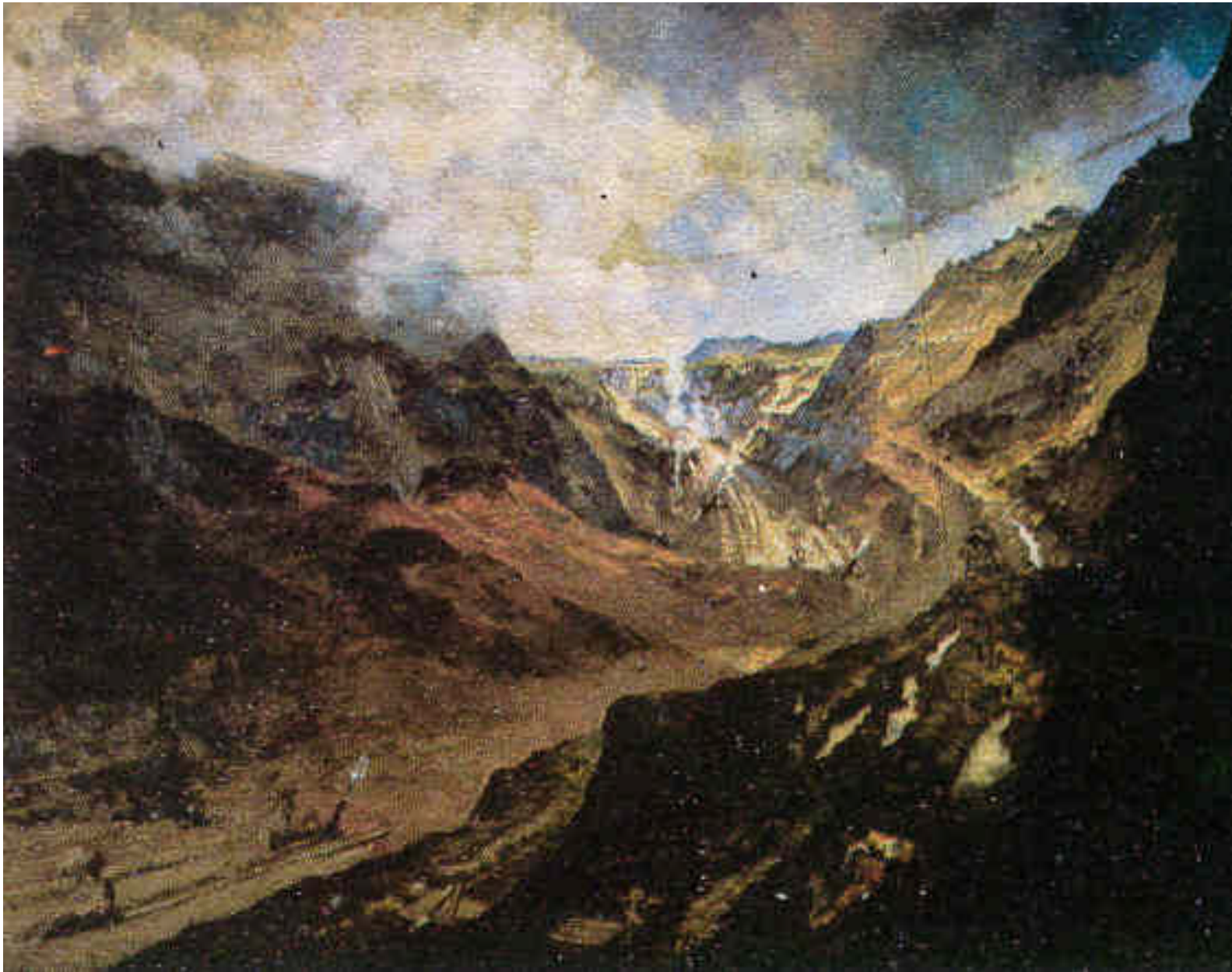
Above: “The digging of Gaillard (Culebra) Cut at Gold Hill”
