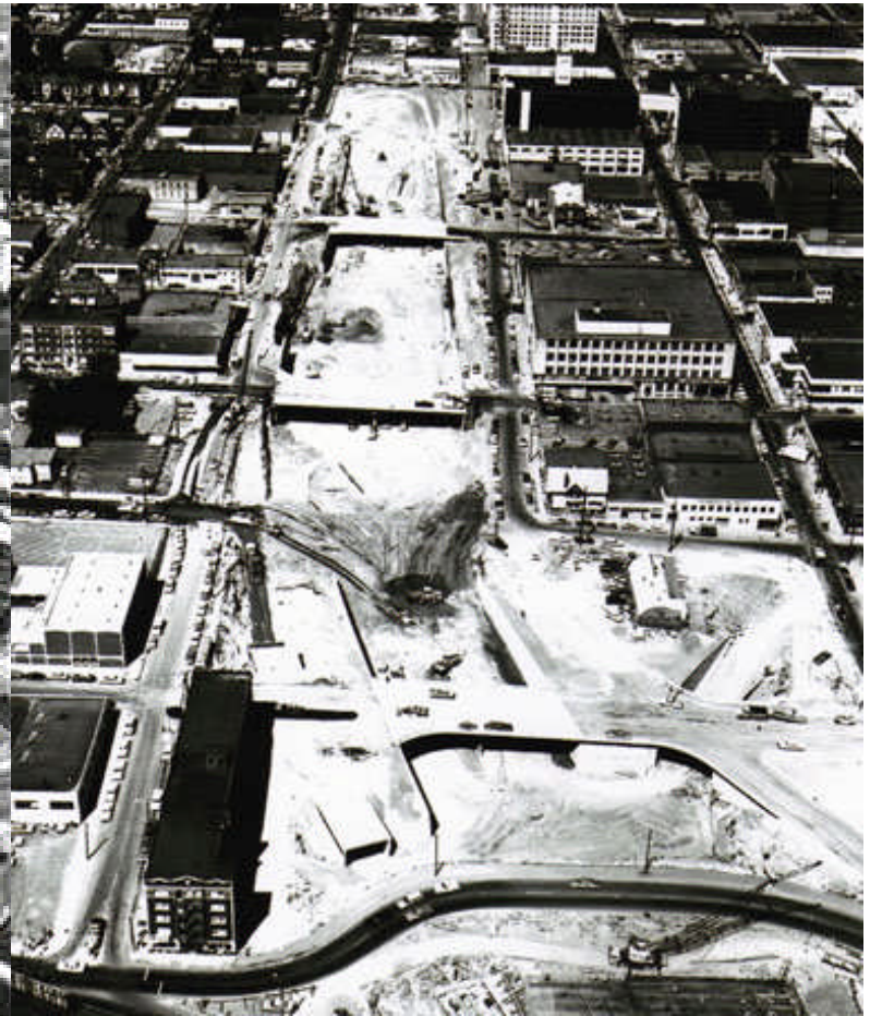
Above: caption: "Oregon - An expensive and difficult project is the construction of the Stadium Freeway (I-405) through metropolitan west-side Portland. Work is well advanced with some of the over crossing already opened to traffic."
