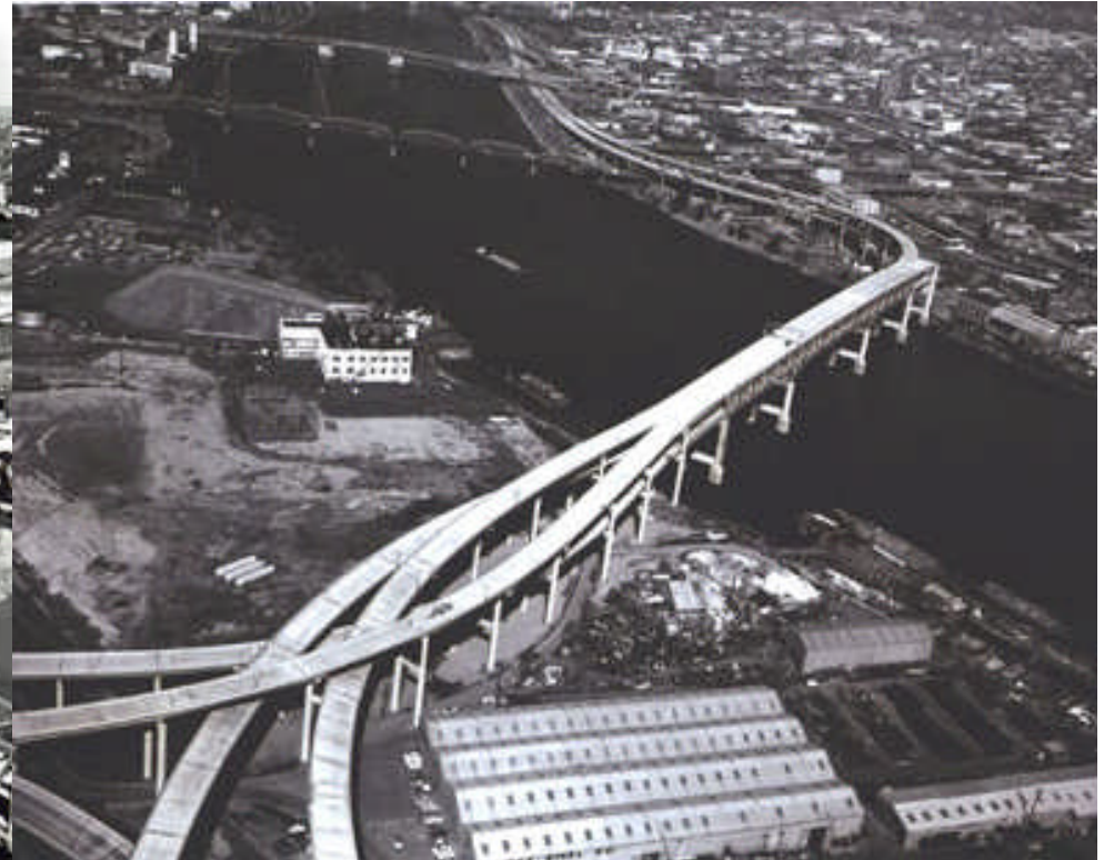
Top Left: caption: “Ohio- Interstate Route 71 & 75 cross the Ohio River from Covington, Kentucky, on this two-level bridge into Cincinnati, Ohio, where ramps distribute traffic to the two diverging Interstate routes and the city Streets.”
