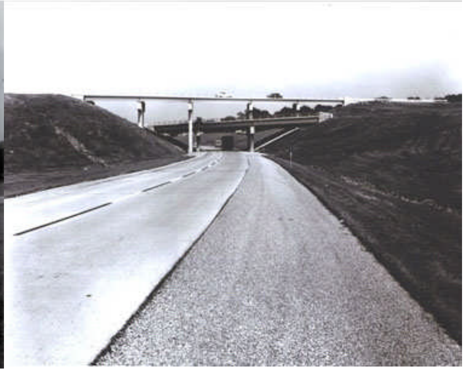
Top Left: caption: “Interstate 94 (Edens Expressway) showing 6 traffic lanes, off ramp right and one ramp left, steel cable guard in median, Chicago, Illinois.”
