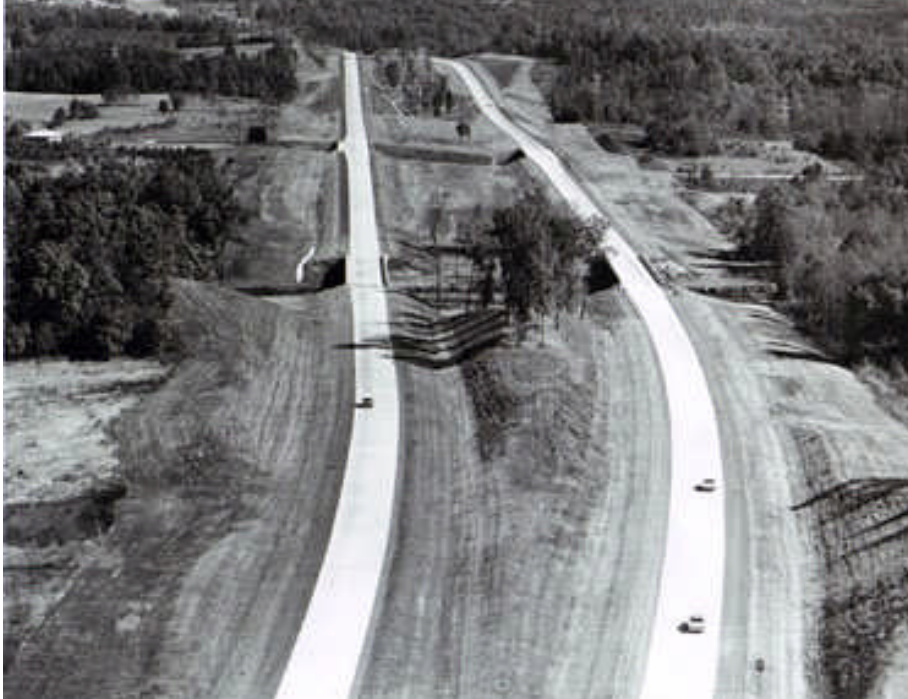
Top Left: caption: “Alabama - Separate roadways fitted into the landscape, as seen beyond the diamond interchange, are typical of design on Interstate Route 59 between Argo and St. Clair Springs.”
