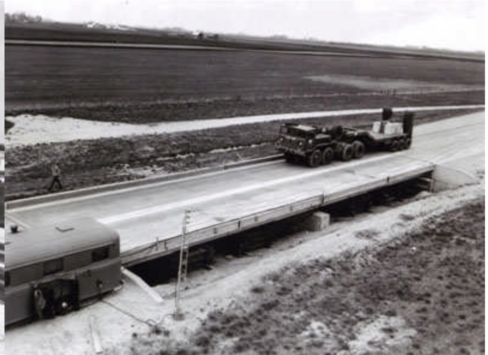
Above L&R: caption: “AASHO Road Test Illinois - Traffic over Test Bridge.”
