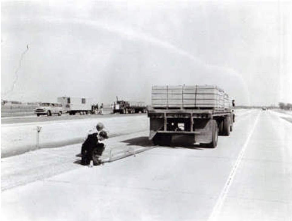
Above L&R: caption: “AASHO Road Test Illinois - Traffic over Test Bridge.”
