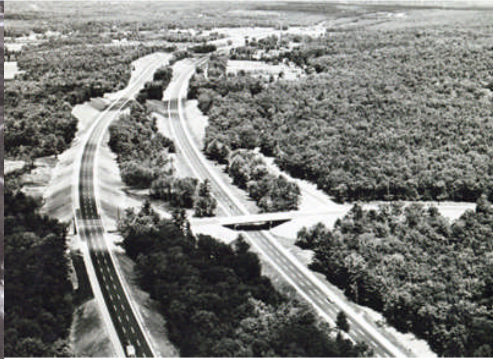
Top Left: caption: “Alabama - Separate roadways fitted into the landscape, as seen beyond the diamond interchange, are typical of design on Interstate Route 59 between Argo and St. Clair Springs.”
