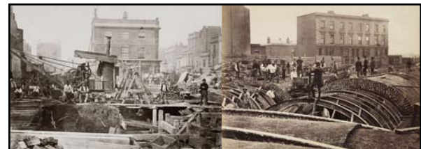
Left: one of a series of photographs by Henry Flather showing the construction, undertaken between 1866 and 1870, of the Metropolitan District Railway's underground lines between Farringdon and Paddington and on to Kensington. It now forms part of the existing District and Circle Line/s on the London Underground. The construction work, utilizing the cut and cover technique, caused a lot of disruption to London neighborhoods. Praed Street station (now known as Paddington), is hidden from view by the beer house in the center of the picture.
