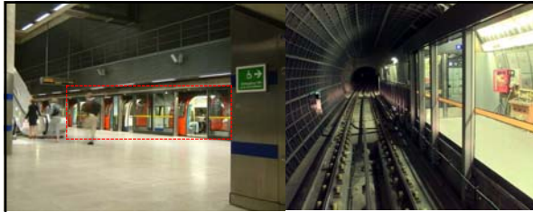
Left: train stopped at Canary Wharf Underground station. The platform-edge doors (outlined) were primarily introduced to prevent drafts underground and to assist in air flow. They also prevent people from falling or jumping onto the track. Right: part of the new Jubilee Line Extension is seen at Westminster station, with platform edge doors (at right)
