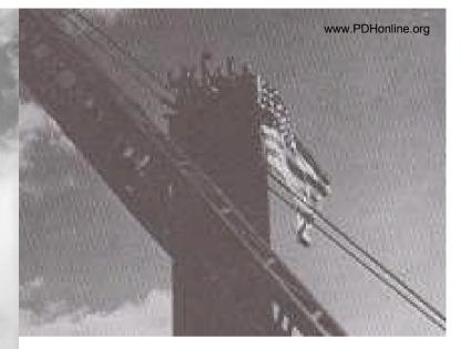
Left: caption: "Tower fully erected (though not fully riveted) with 80 foot booms to handle materials atop." <u>Above</u>: caption: "Finally, on October 22, 1955 the first topmost piece of steel was erected, and according to tradition Old Glory waved proudly with the men who put it there, 552 feet above the Straits."
