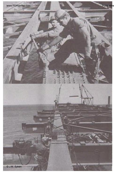
Top: caption: "Bridgemen tightening high tension steel bolts used for all truss span connections. Meter in torque wrench must be carefully observed to make sure that a bolt is neither too tight nor too loose. Every bolt was inspected."
