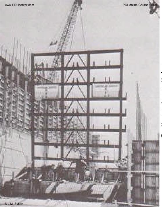
Left: caption: "This threestory high chunk of steel is called an 'Anchor Bar Support Frame,' and that is just what it does: support the anchor bars (Pier 22)."
