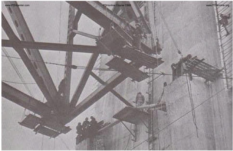
Above: caption: "A close-up shows there were about six feet to go before the backstay span lined up with the steel shoe into which it 261 would eventually fit." 261
