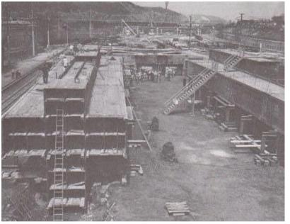
Left: caption: "Meanwhile the towers were not only being fabricated but were being built – horizontally instead of vertically – some 500 miles from the Straits of Mackinac. At Ambridge, Pennsylvania, the towers were laid out on the ground and drift-pinned together to see if all parts fit properly. This picture showing the bottom section provides a clue to their enormous size." **PDHonline Course C668**
