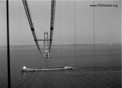
Left: caption: "Storm guys were attached to the catwalk securing it to the towers and the anchor blocks to help resist high winds and storms. The billowing sails of the yacht below complement the curves of the catwalk and highlight the strong winds present in the Straits."
