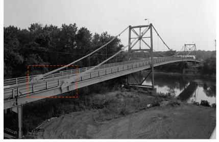
Above L&R & Left: the Hutsonville Bridge (a.k.a. Sullivan-Hutsonville Bridge) connects Crawford County, Illinois with Sullivan County, Indiana over the Wabash River (built in 1939 and replaced in 1988). It was a rare example of the self-anchoring suspension bridge type (above L&R).
