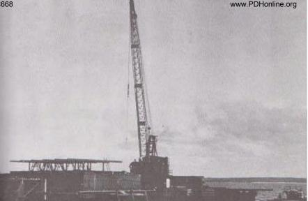
Left: caption: "The Pier 18 caisson, 44 x 92 feet, was assembled at Toledo to a height of 38 feet. It was towed to the Straits, positioned in its corral, and the process of driving it to rock bottom was the same as for the circular caisson. Here another lift of digging wells and wall is being welded to the top of the caisson."
