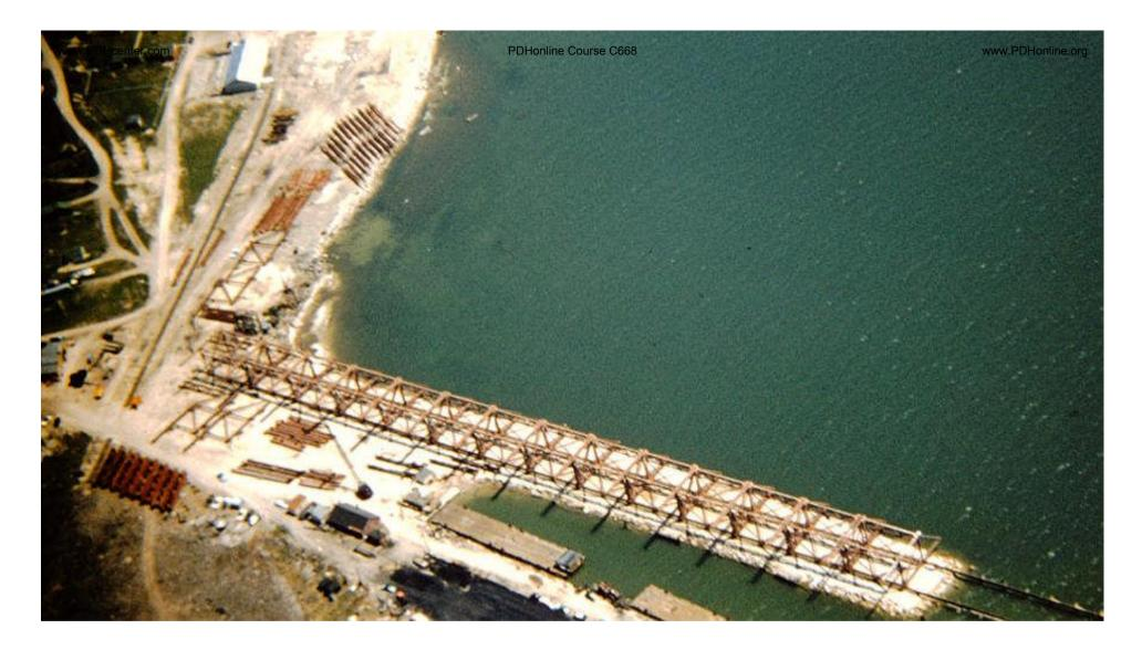
Above: caption: "Mackinac Bridge truss spans being assembled on shore before being towed into position and raised into place." 307
