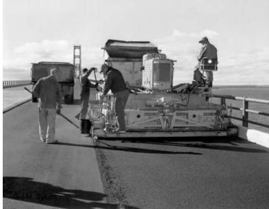
Above: caption: "Deck contractors pulled out all the stops to complete the concrete roadway all the way out to the cable-bents where the steel and lightweight concrete roadway begins."
