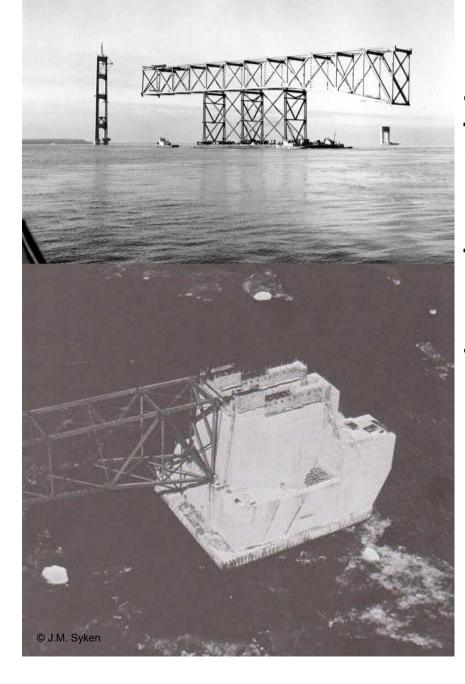
**Top:** caption: "North backstay span under tow to site. December 18, 1955." **Bottom:** caption: Exactly the same operation was performed on December 18, 1955 to place the north backstay span, shown here with the north anchor block as winter weather moved in (Pier 22)."
