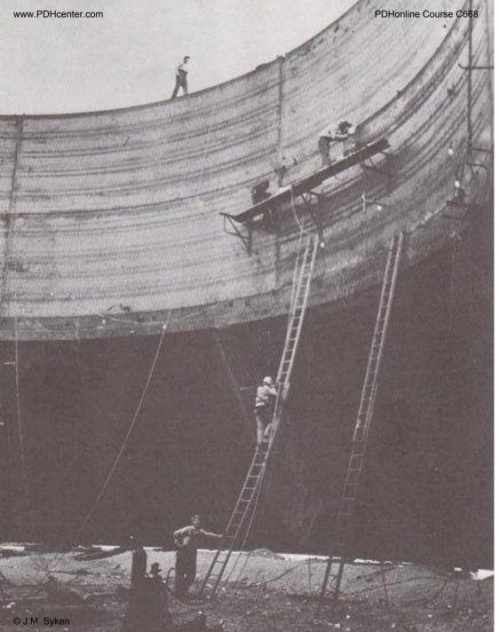
Left: caption: "Inside the caisson, welders sealed all parts so that it became watertight between the walls. These were then divided into eight watertight compartments (Pier 20)."
