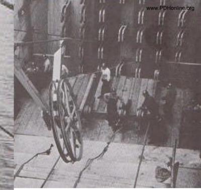
Left: caption: "A bridgeman walks the double-grooved spinning wheel from anchorage to ascertain that it is properly working before the machinery is pressed into action."
