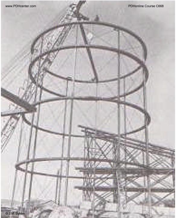
Left: caption: "The steel framework for one of the pair of cofferdams took shape on land at St. Ignace. One of the units for a caisson corral is in the background."
