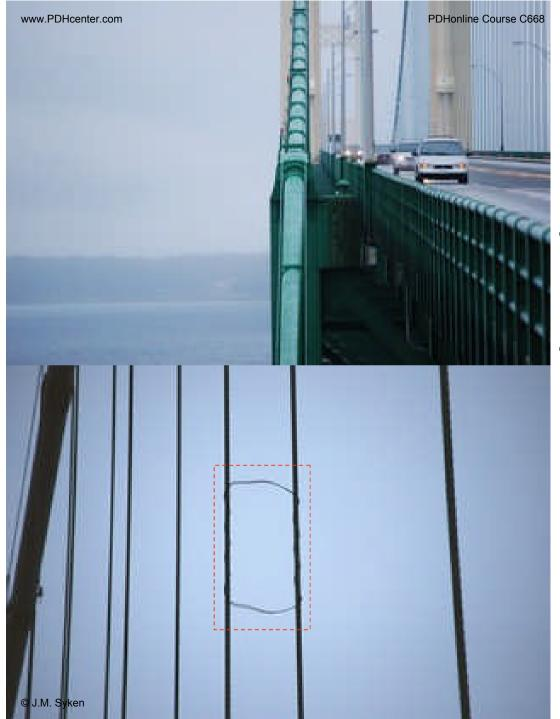
Top: caption: "Bridge cable as seen from top of anchorage" <u>Bottom</u>: caption: "Horizontal wires between cables keep cables from hitting each other during strong winds."
