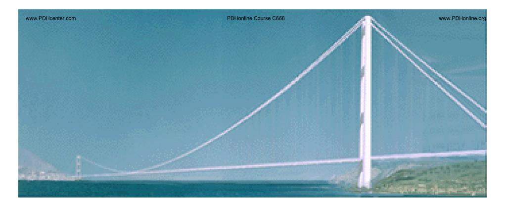
"...The Steinman design for the Messina Straits Bridge has been replaced with a design for an even longer span that incorporates later developments in suspension bridge technology, but some of his legacy remains in the current design for a 3,300m span: e.g., in the use of a partially open grid deck to improve aerodynamic performance..." Maria Grazia Bruschi, Structural Engineer
