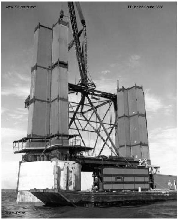
Left: caption: "Using the creeper derrick to erect the fourth tier of the Mackinac Bridge north tower. This ingenious device mounted with a boom raised steel and climbed up the steel it raised. August 9, 1955."
