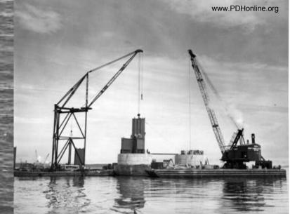
Above: caption: "North Mackinac Bridge tower. Placing steel section, 2nd tier, west leg. July 5, 1955"
