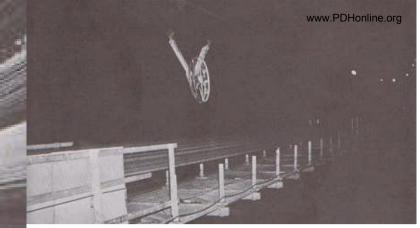
caption: "While Left: spinning was taking place on one cable, bridgemen adjusted, squeezed and handled the strands on the other." Above: caption: "Cable spinning was carried on in two ten-hour shifts so long as weather permitted."
