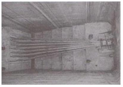
Left: caption: "By the end of October the cable splay area chamber was complete. The cable enters the anchor block, at right, through the cable saddle. The multiple strands of the cable then disperse, like the roots of a tree. Looped around a strand shoe, each cable strand is securely attached to an exposed end of a deeply embedded eyebar, left."
