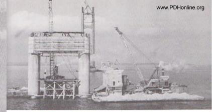
Left: caption: "A massive steel arch was raised to the top of the concrete towers and made a bridge connecting them." <u>Above</u>: caption: "Forms were built around the arch frame, and they were filled with concrete."
