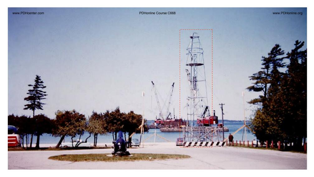
Above: construction of the Mackinac Bridge officially began on May 7<sup>th</sup> 1954 at what was the parking lot for Michilimackinac State Park. The metal structure (highlighted) was one of seven land-based survey towers at fixed locations which were used along with six waterbased towers. By sighting along lines from one location to another and by directing surveyors in boats to position themselves where these lines crossed, the location/s of piers was thus determined precisely.
