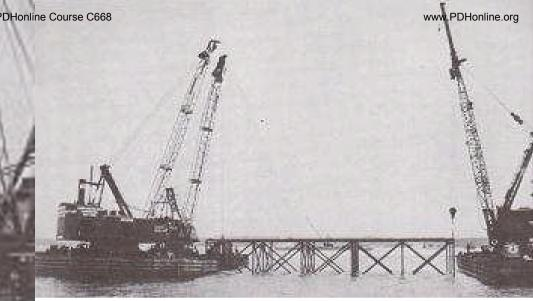
Above: caption: "When in position, the steel frame was picked off the barge by three marine cranes, sometimes called 'whirlies' because they turn a full circle, and gently lowered to the overburden. This is the sand, mud, clay, broken stone and miscellaneous soft material lying under water and above bedrock."
