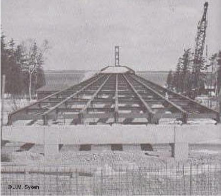
Above: caption: "On the north side the connection from the bridge deck to the causeway level was started with the completion of 14 bents on which steel and roadway would be built."
