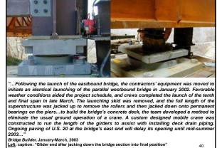
zuos... <u>Left</u>: caption: "Glider end after jacking down the bridge section into final position" <u>Right</u>: caption: "Jacking girders down onto permanent bearings"
