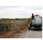
Left: caption: "Spraying hydroseed on exposed soil along new access road. Hydroseed consists of seed, ground paper or wood fiber and water. The mixture is sprayed on and forms a crusty coating that anchors the soil until the seed can germinate."
