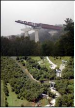
"The trick was always to have enough weight behind the support so the bridge won't tip over as you push it. You're applying a force of 800 kips on the back end of the bridge, and you've got a snake of steel 1,500 ft. long and you're trying to keep it corralled in a straight line...It was a big relief to get past the first launch. There were a lot of nervous people that day. If a launch had ever overshot the next pier, there was no way to back up.
