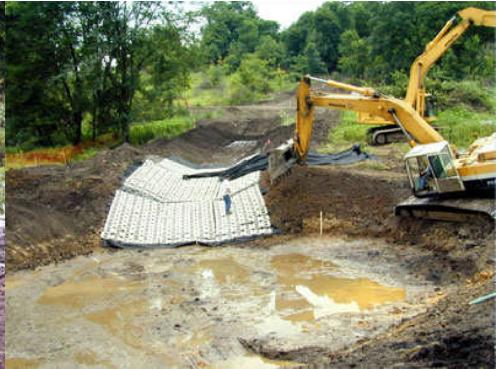
Top Left: caption: “Installation of the cable-concrete panels to prevent erosion”
