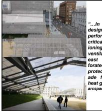
"...In the tower, the design of the highperformance facades is critical to the functioning of the natural ventilation. At the southeast elevation, a perforated metal sunscreen protects the glass facade from excess solar heat gain..." arcspace
