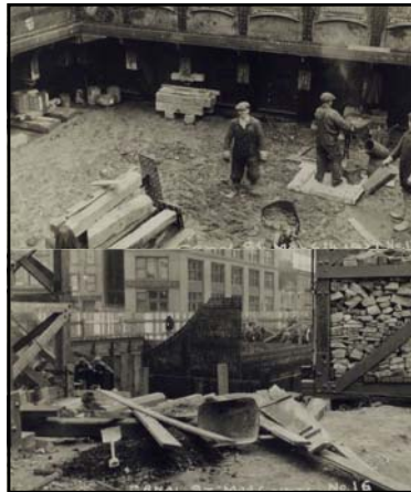
Top: caption: "Working chamber, Cutting edge, Blocking. Canal Street, May 6, 1921"
