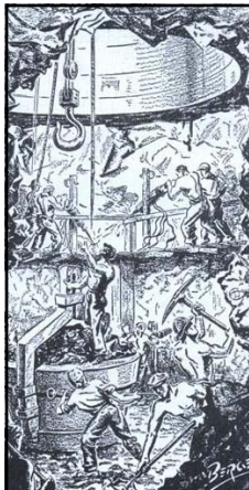
Left: caption: "Artist's drawing: sinking of the preliminary shaft"
