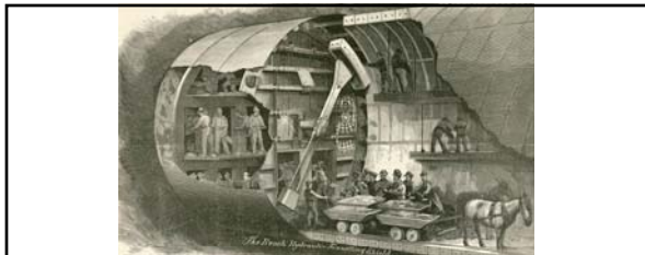
"...The modern tunnel shield is a steel-plate cylinder whose forward edge acts as a cutting edge. Its rear end, extending backward, overlaps the tunnel lining of cast-iron rings. Inside the shield, hydraulic jacks act against the tunnel lining as a thrust block so as to push the shield ahead when pressure is applied. A partition prevents earth from entering the shield except as permitted through suitable openings. As the shield moves forward, the lining is erected under the protection of its rear. In submarine tunneling compressed air pumped into the forward end of the tunnel counter-balances the pressure of the water which tries to enter..."
