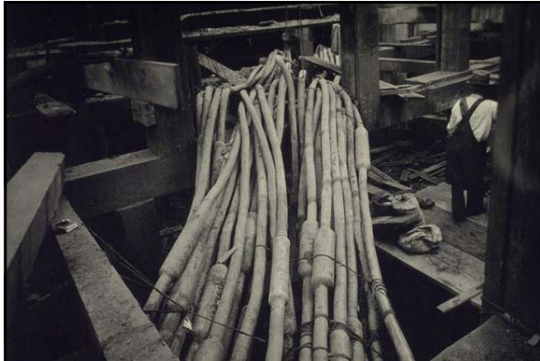
Above: caption: N.Y. Telephone Co. cables at Canal & Hudson Streets, New York. 12/2/24. 115
