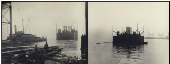
Right: caption: "...River-shaft caissons were built, launched, floated into position, and sunk, as on the New York side..."
