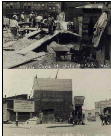
Top: caption: "Concreting, mixing plant. Canal Street, July 14, 1921"
