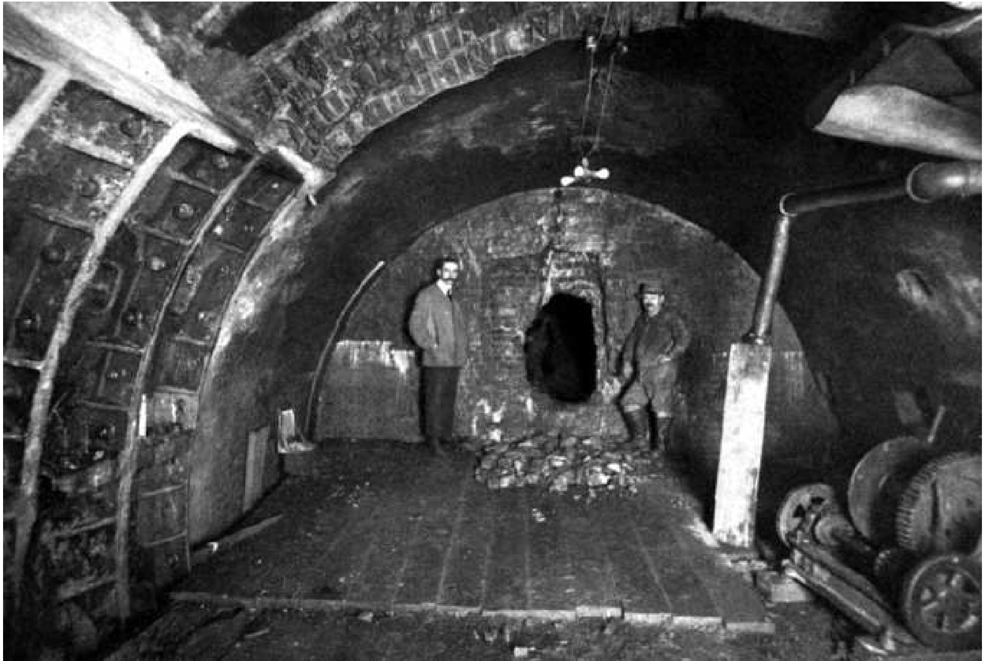
Above: caption: “The south tunnel holed through, breaking into the brick bulkhead at the Morton Street shaft. The newly completed tunnel is in the foreground.” 157
