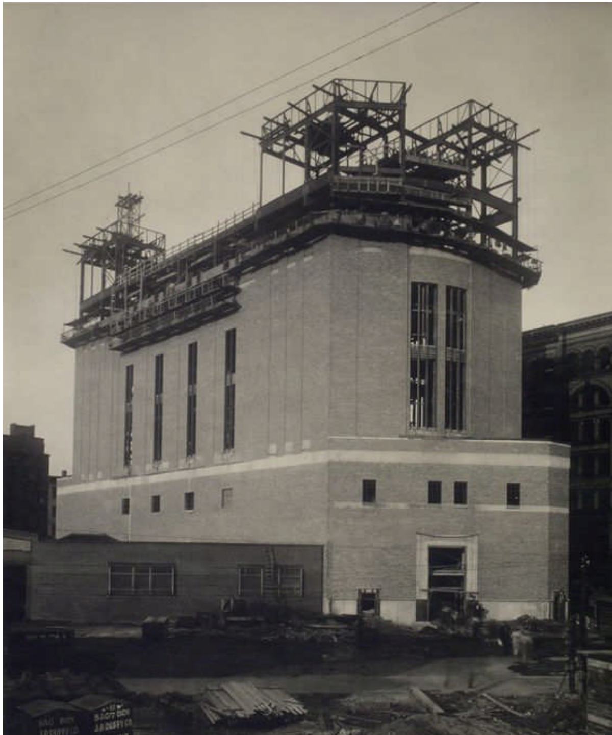
Left: caption: “Brick work - Land Ventilation Building. North side of Canal Street, west side Washington Street, New York. 10/7/26.”
