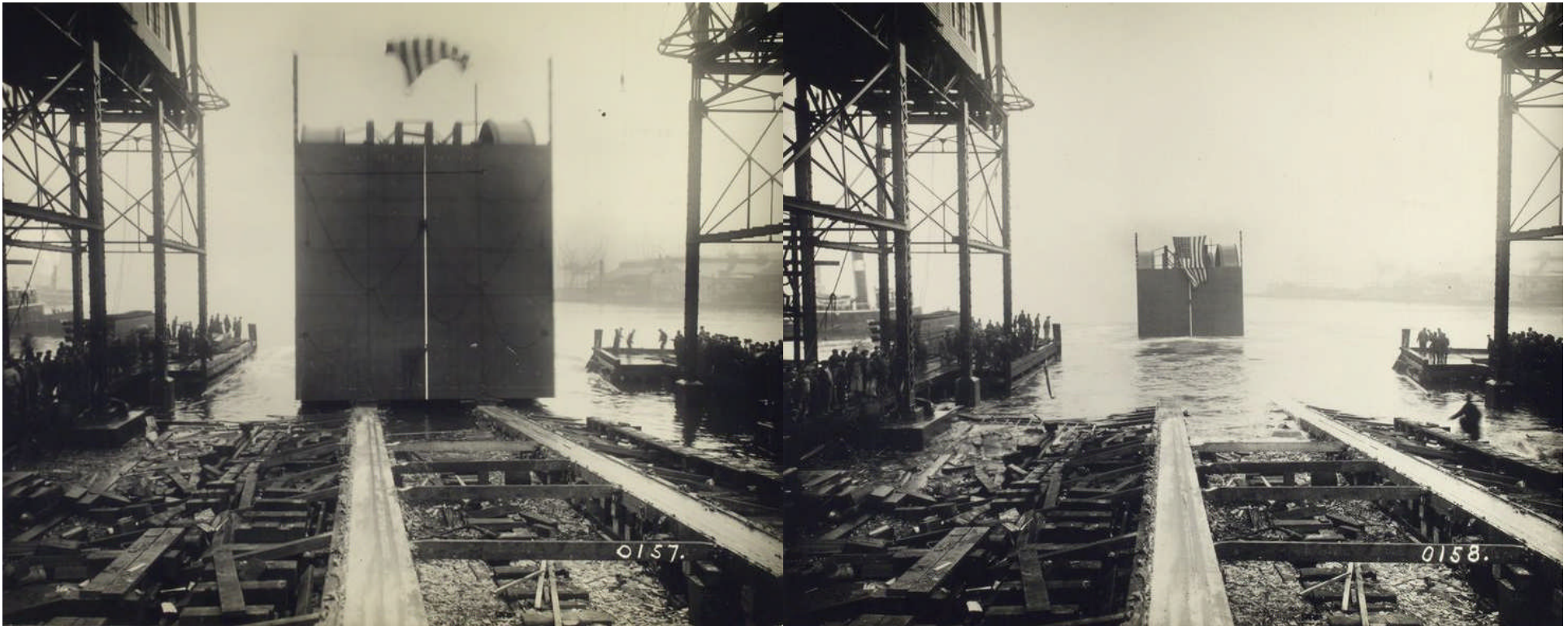
Above L&R: caption: “View of launching of New York River Shaft Caisson, Staten Island Shipbuilding Co.’s Plant, Mariner’s Harbor, S.I. 12/5/22.”
