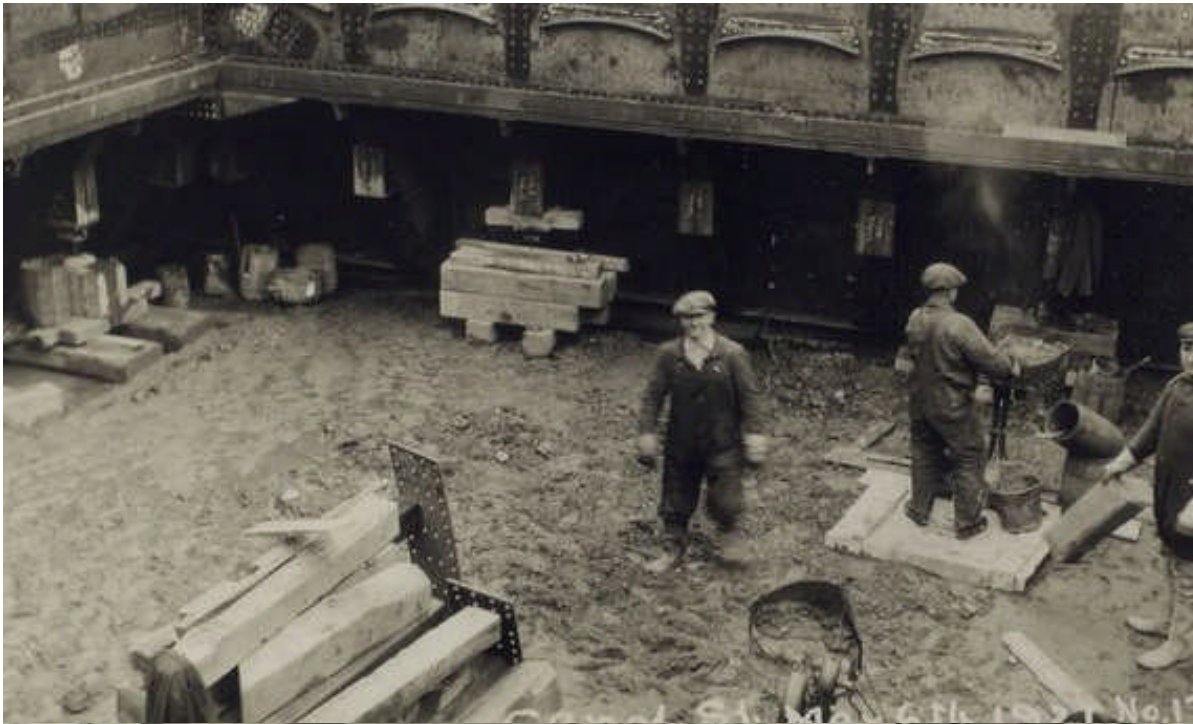
Top: caption: “Working chamber, Cutting edge, Blocking. Canal Street, May 6, 1921”
