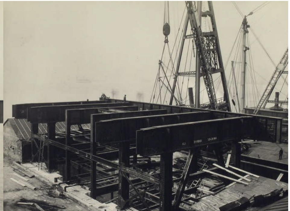
Above L&R : caption: “River Ventilation Building, New York. Erection of steel girders. 3/12/26.”
