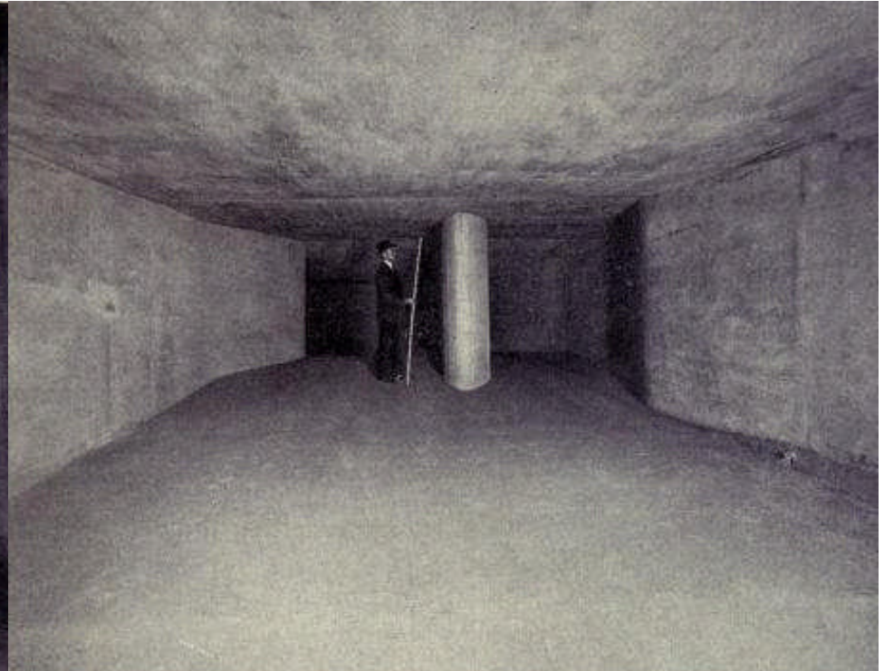
Top Left: caption: “East Blower Air Duct. In Land Ventilation Building, New York City, showing curved back and vanes.”
