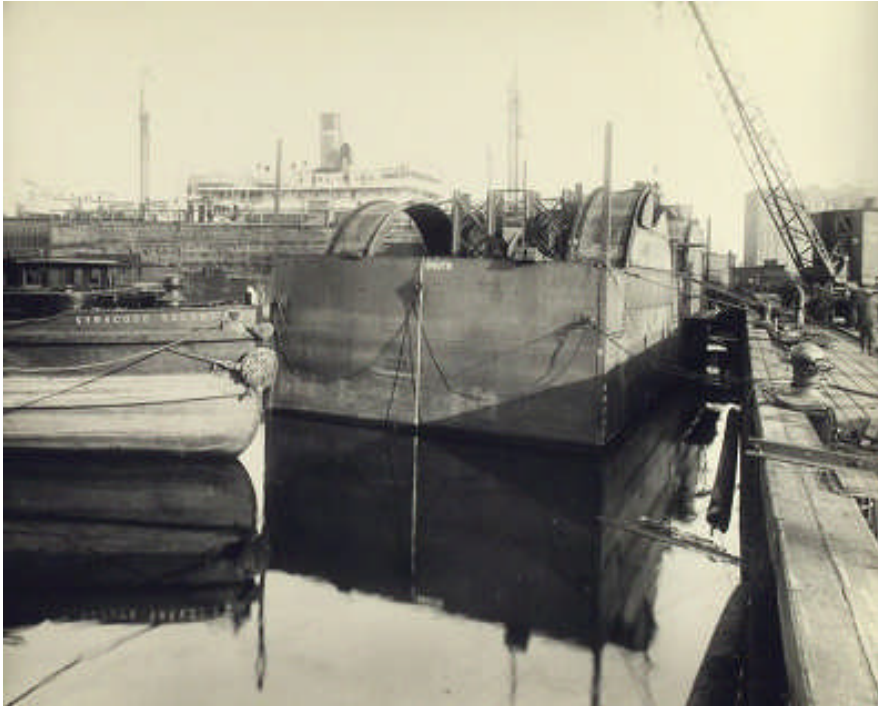
Top Left: caption: “View of launching of New York River Shaft Caisson, Staten Island Shipbuilding Co.’s Plant, Mariner’s Harbor, S.I. 12/5/22.”
