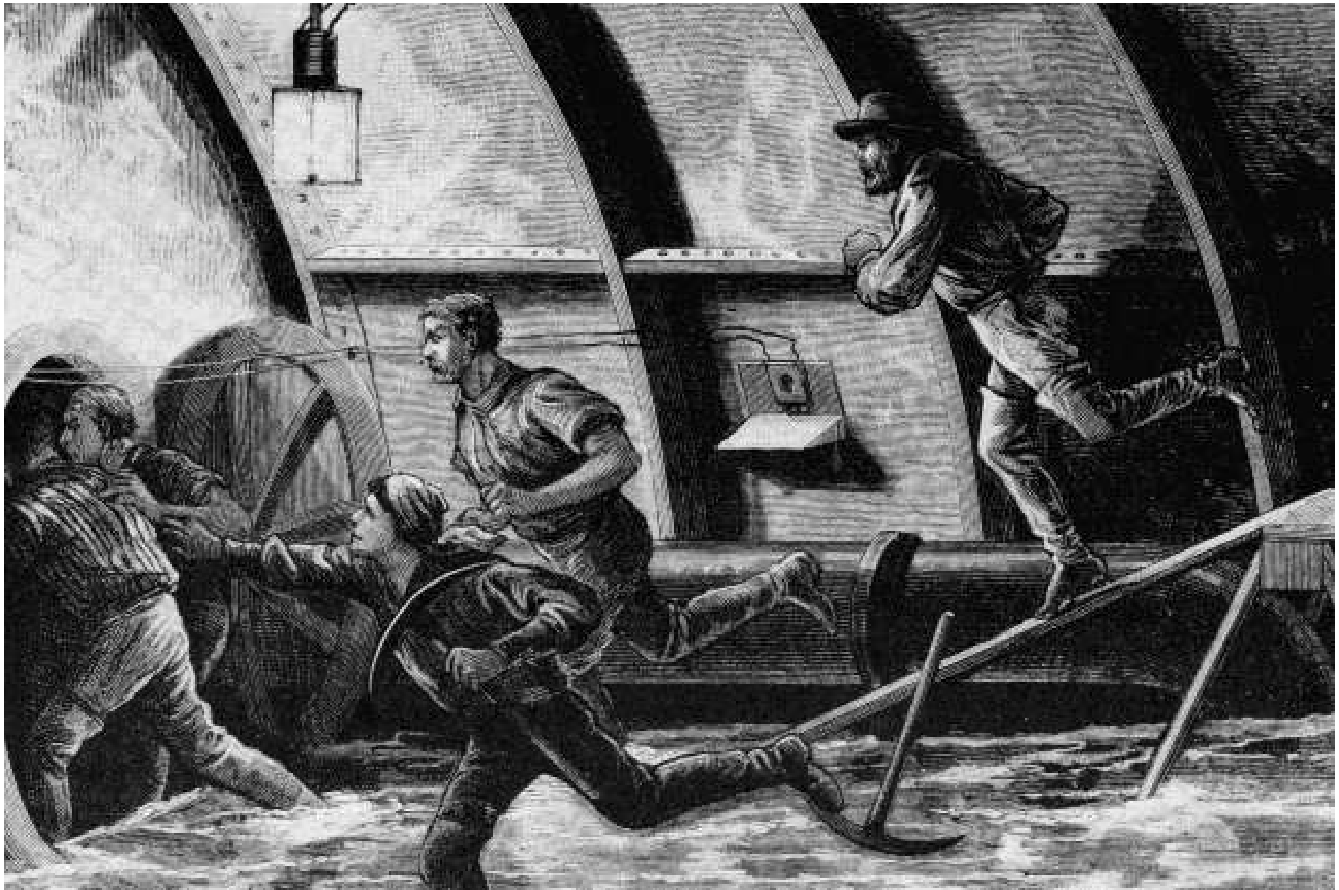
Above: caption: “Artist’s conception of miners escaping into the air lock during the blowout in Haskin’s tunnel”
