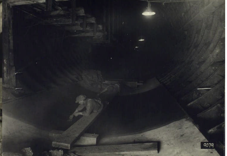
Above Top: caption: “Steel pile segments and forms for setting concrete invert. 4/30/25.”
