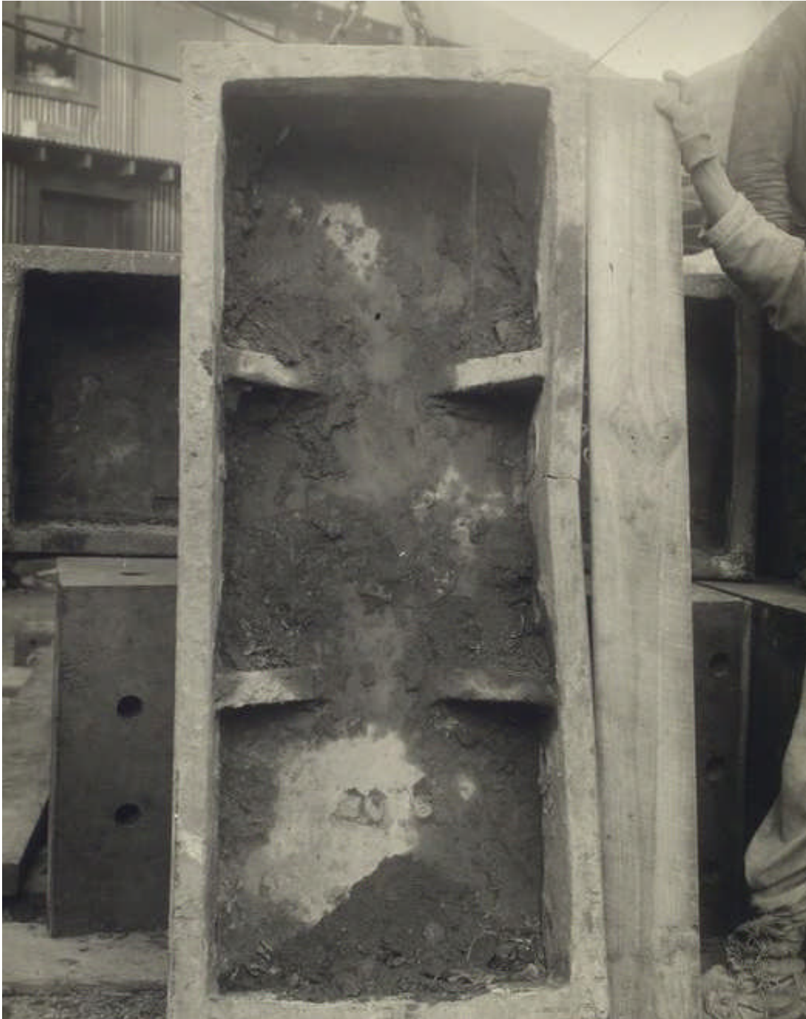
Above & Left: caption: “Broken plate. Cast- iron lining South tun- nel. 11/22/22.”
