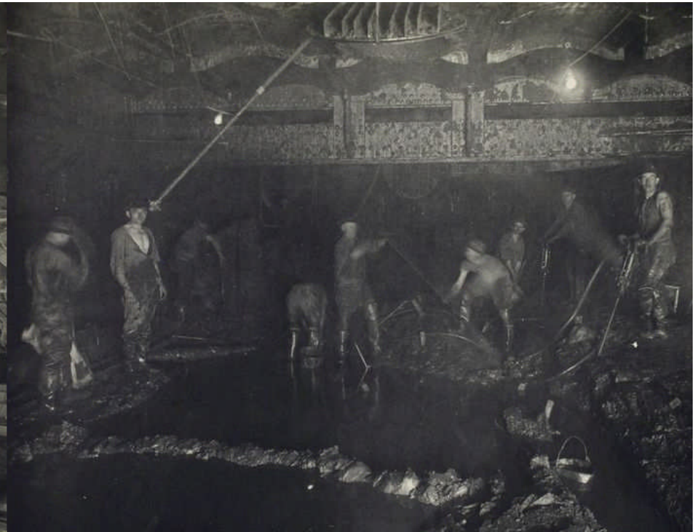
Top Left: caption: “General interior, view of working chamber, New York River Shaft Caisson. 12/20/22.”
