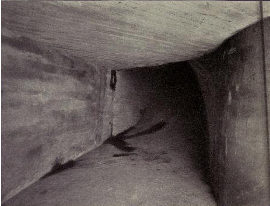
Top Left: caption: “East Blower Air Duct. In Land Ventilation Building, New York City, showing curved back and vanes.”
