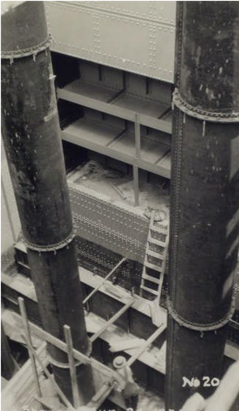
Above: caption: “General view. Caisson about ready to start sinking. Concrete chute at left, hoisting engines in front, air lines at side. Spring Street, June 24, 1921”
