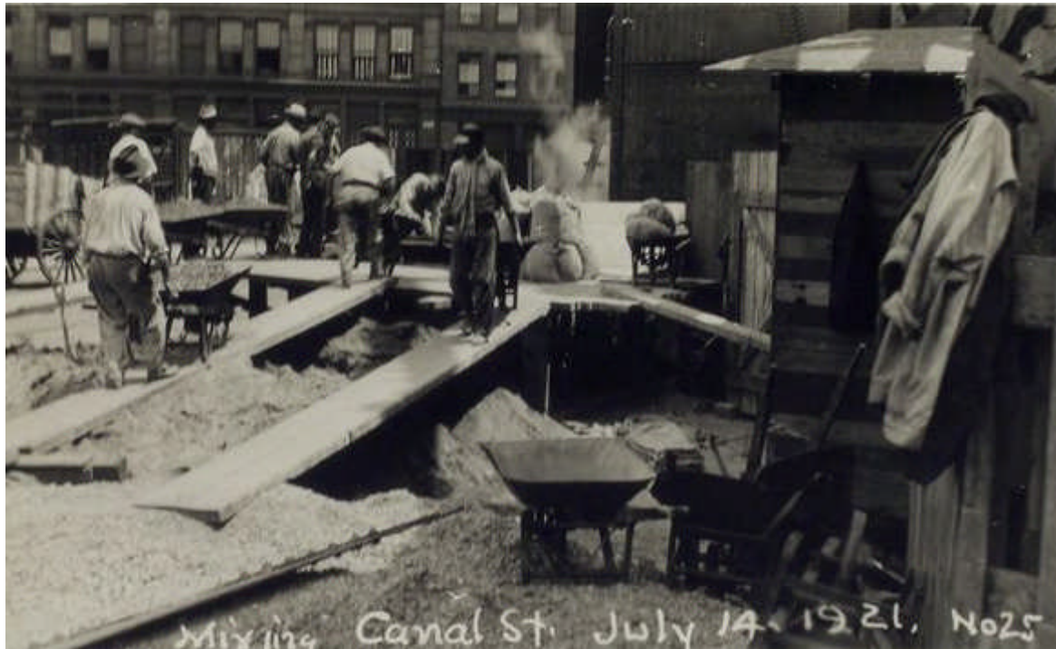
Top: caption: “Con- creting, mixing plant. Canal Street, July 14, 1921”
