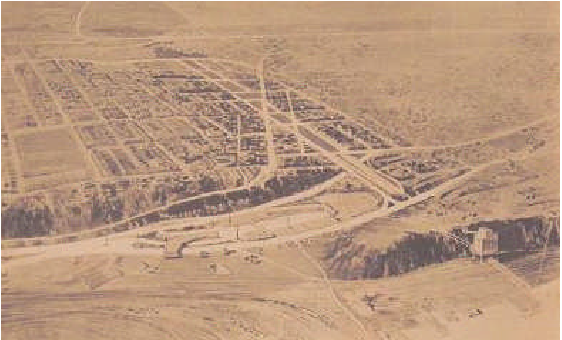
Above: caption: “Initial Arrangement of New Jersey Approach. Weehawken toll plaza with its initial to Hudson County Boulevard East and Park Avenue as completed to form part of the First Operating Unit of Lincoln Tunnel. The uncompleted structure at Hudson County Boulevard East will form part of the viaduct loop which is now under construction.” (as of December 1937)
