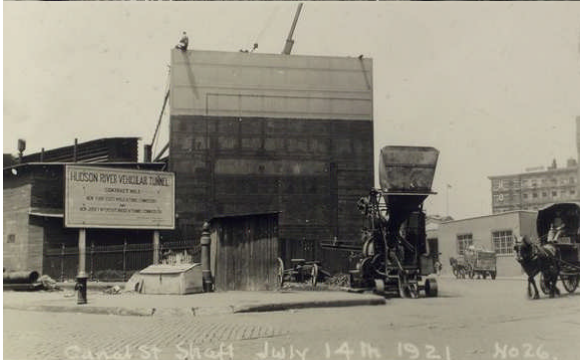
Bottom: caption: “Pai- nting. Canal Street Shaft, July 14, 1921”
