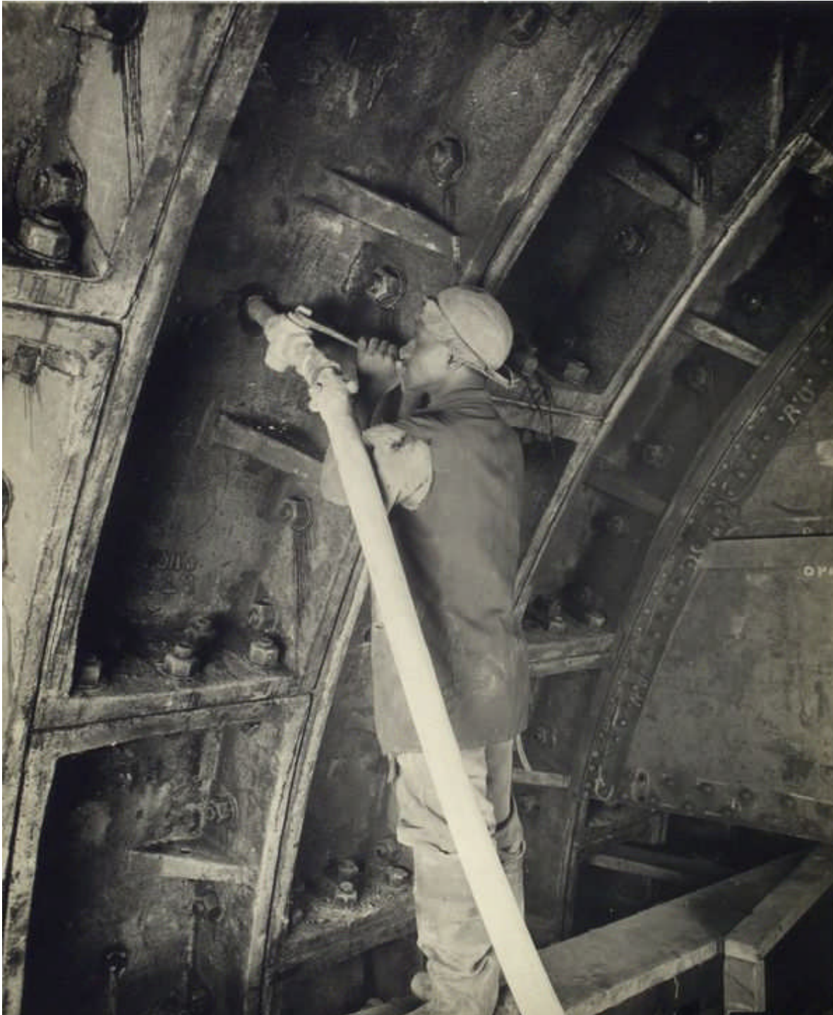
Above: caption: “Grouting in South tunnel, New York. 4/10/23.”
