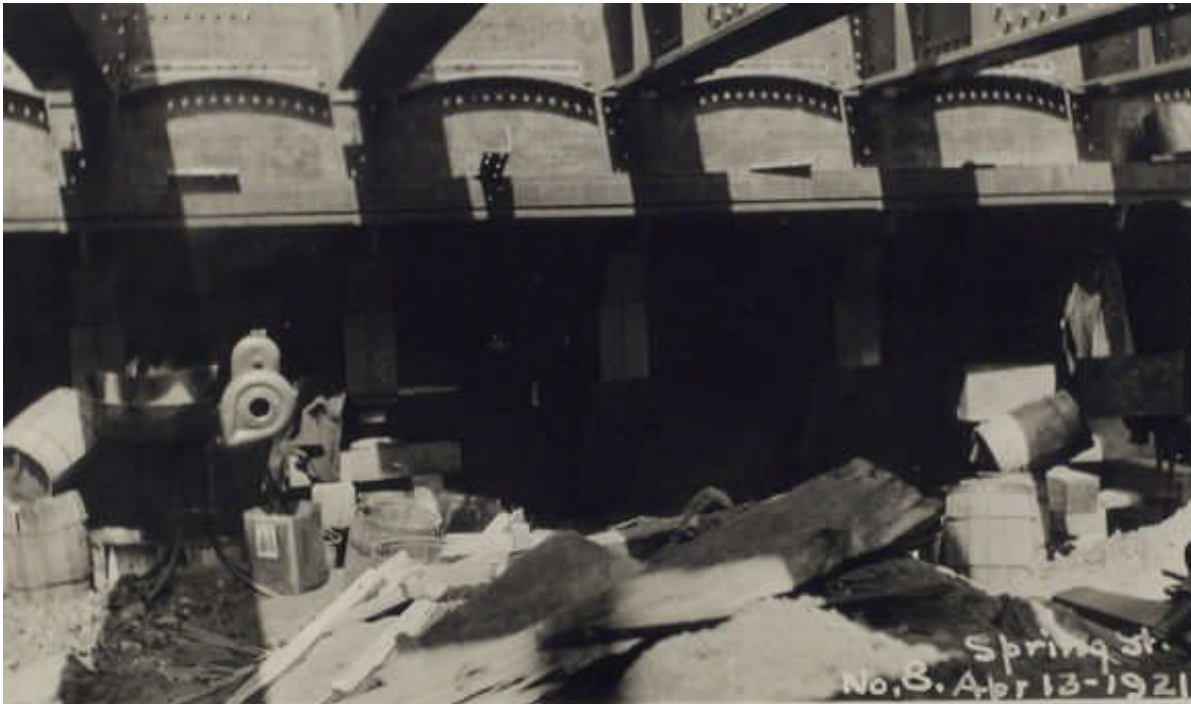
Top: caption: “Working chamber, roof girders bolted. Spring Street, April 13, 1921”
