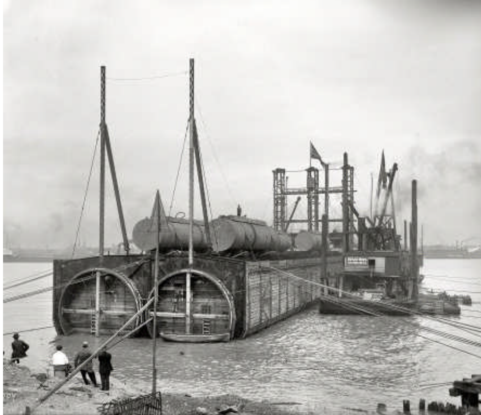
Top Left: caption: “Launching of a section of the Detroit River Tunnel at the Great Lakes Ship Yard St. Clair”
