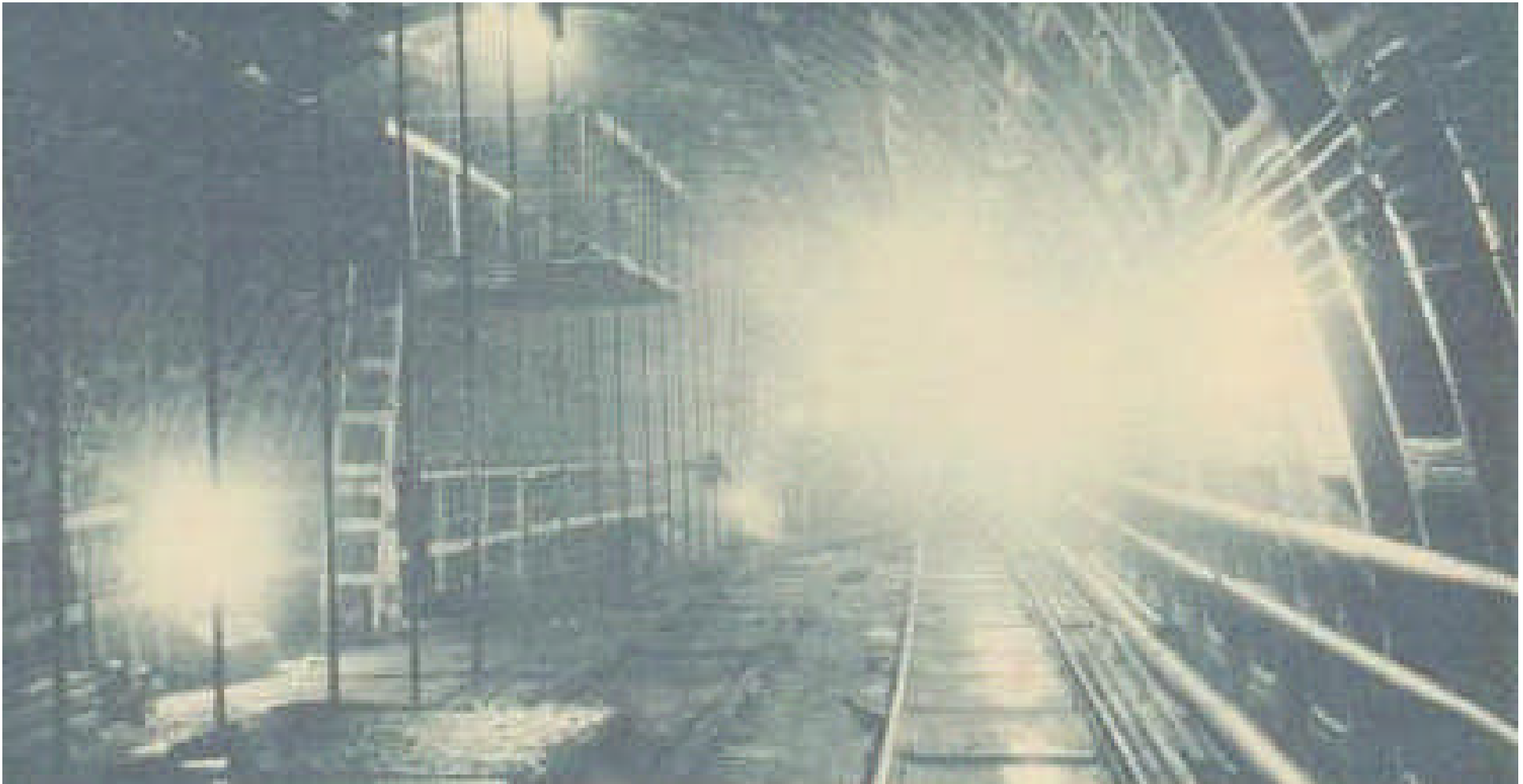
Above: caption: “A great roadway for the motorist of 1938 begins to assume form in the mud and rock of the Hudson River bed: a view in the new Midtown Hudson Tunnel, which has advanced about 200 feet from the New Jersey side of the river and about 600 feet from the Weehawken Terminal Point. The daily movement toward the middle of the river is about twenty-five feet, and great rings of steel are set in place at regular distances for the frame of the tunnel.”
