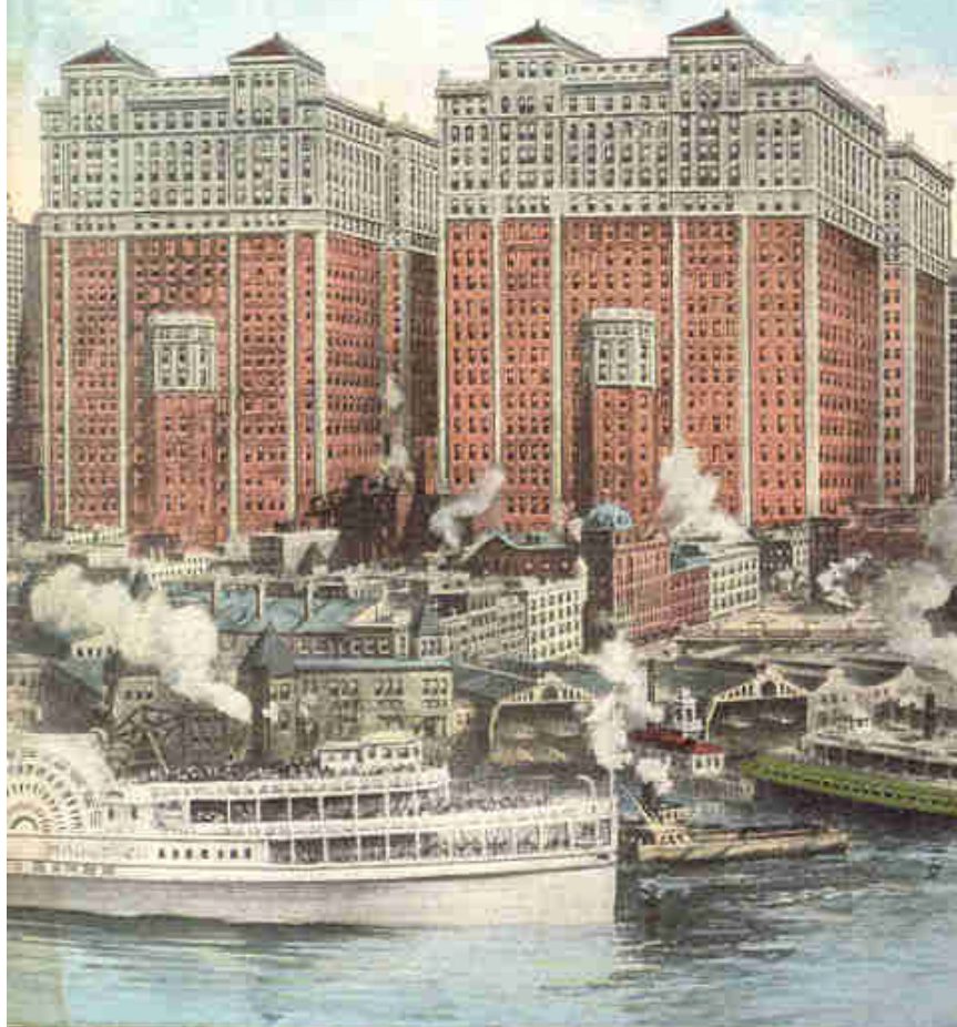
Hudson Terminal and Tubes. New York City.
