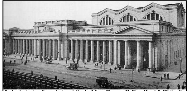
"...In designing the exterior of the building, Messrs. McKim, Mead & White, the architects, were at pains to embody two ideas: To express in so far as was practicable, with the unusual condition of tracks below the street surface and in spite of the absence of the conventional train shed, not only the exterior design of a great railway station in the generally accepted form, but also to give to the building the character of a monumental gateway and entrance to a great metropolis..." RE: excerpt from The New York Improvement and Tunnel Extension of the Pennsylvania Railroad 122
