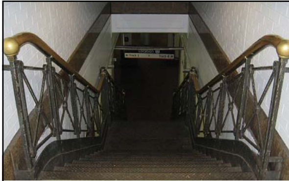
Above: one of the last remnants of the original Penn Station; a staircase between Tracks 3 and 4
