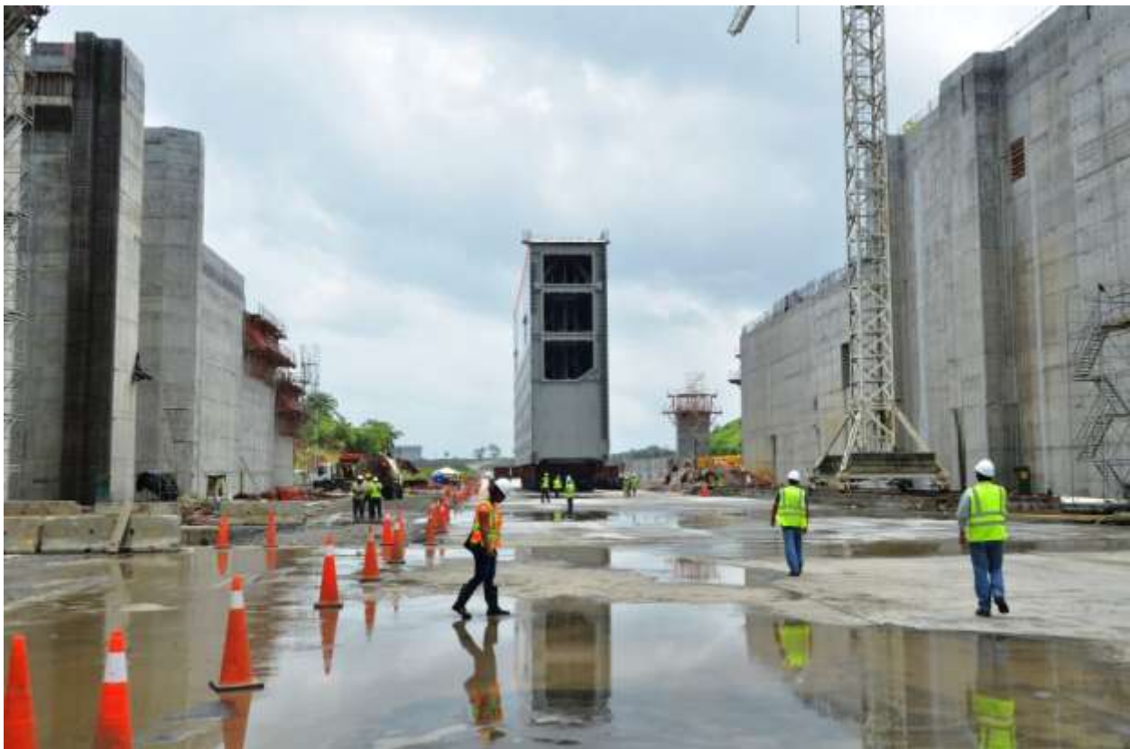
First Gate travelling down a special made highway to the locks
