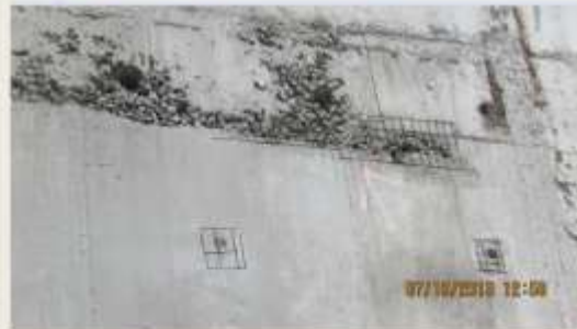
Atlantic Site Voids and Honeycombs in Valve Structures, Backfill and WSB Conduits
