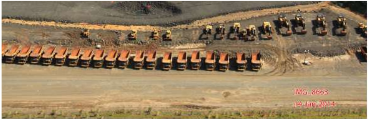
PHOTO PAC 52 - 87 Borinquen Dam 1W - Sector D6 to S
