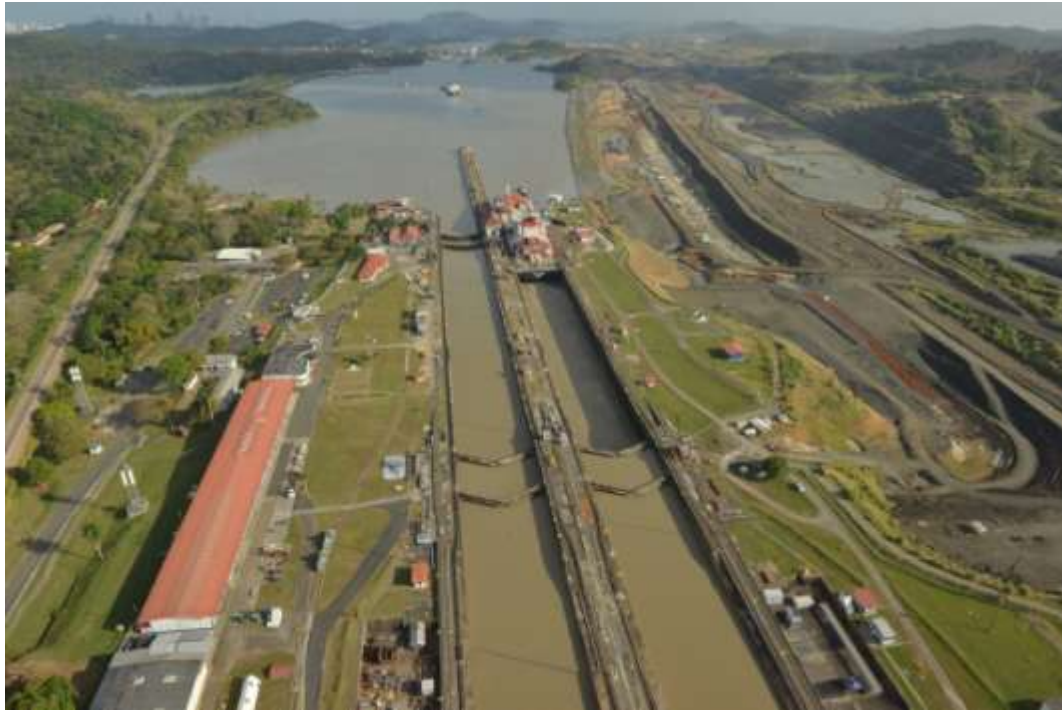
Existing Miraflores lock structure with Borinquen Dam on right
