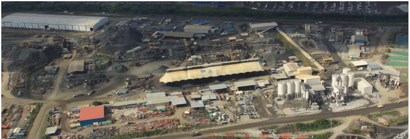
Pacific Site Batch Plant, Crusher Plant, Rebar Fab Shop and laydown areas
