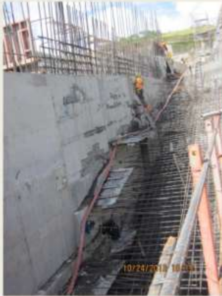
Atlantic Site Voids and Honeycombs in Valve Structures, Backfill and WSB Conduits
