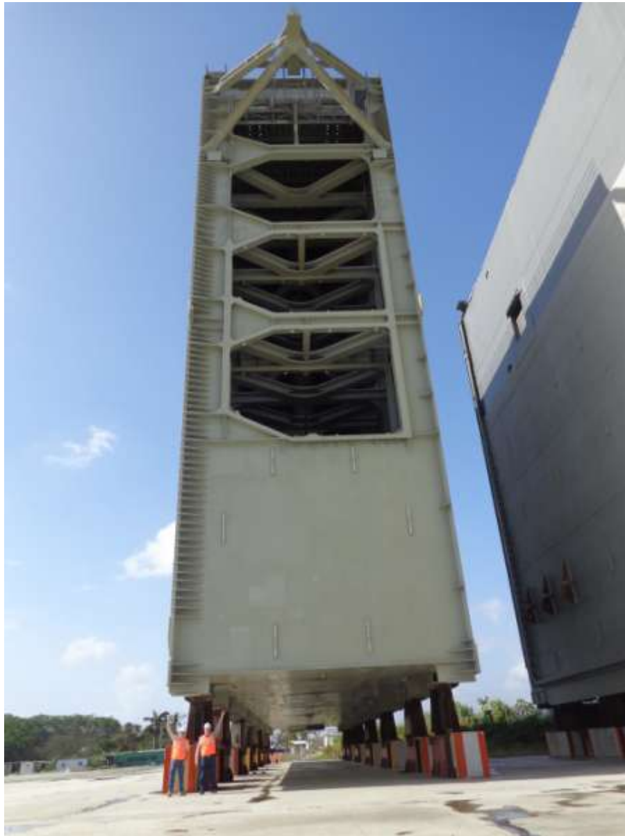
Sliding Gate in laydown on site
