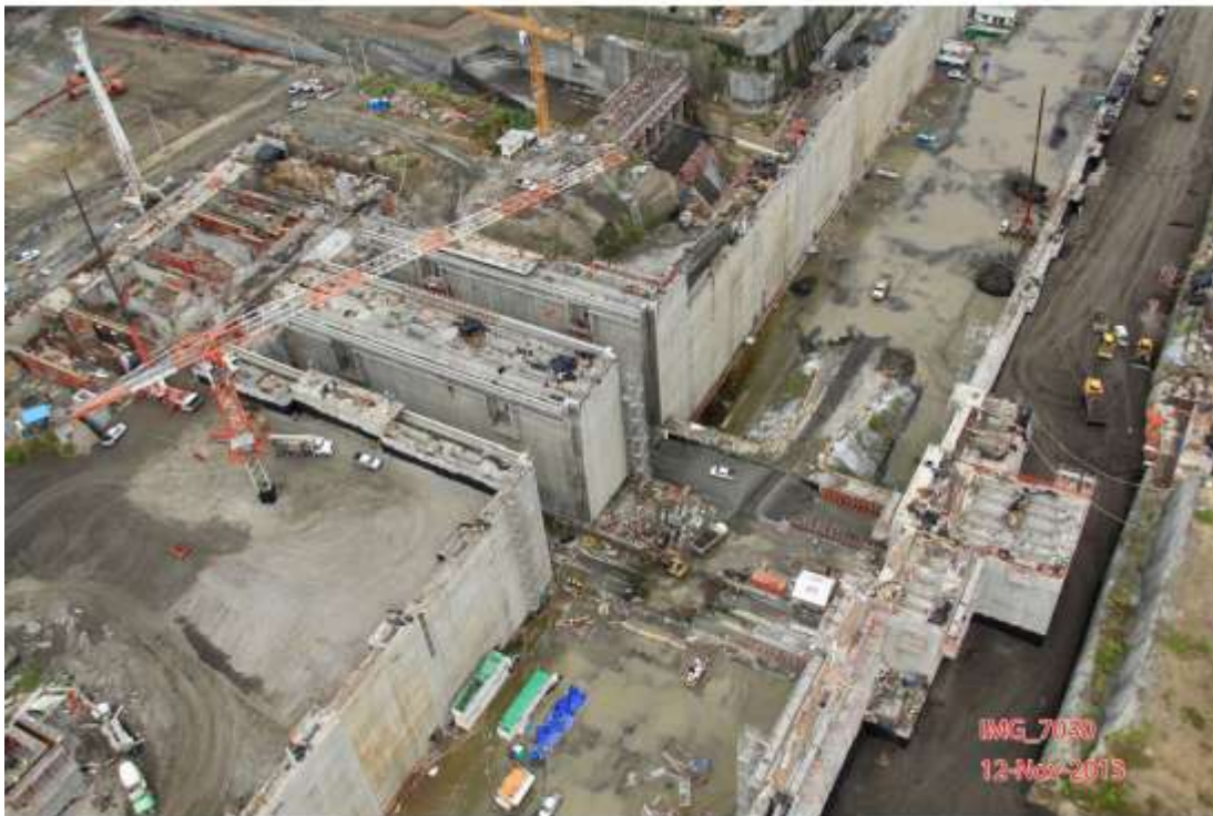
ATLANTIC - LHZ & BACKFILLING
