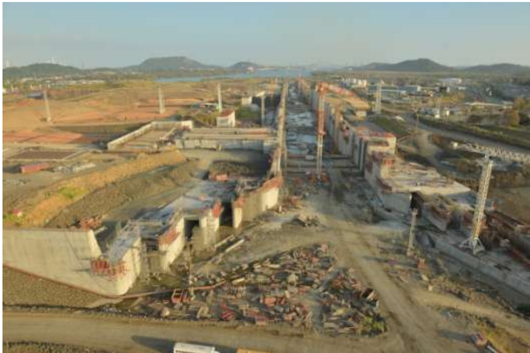
Atlantic Site looking South through the canal chambers
