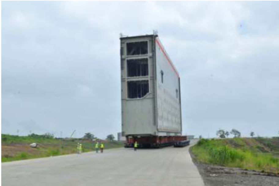
First Gate travelling down a special made highway to the locks
