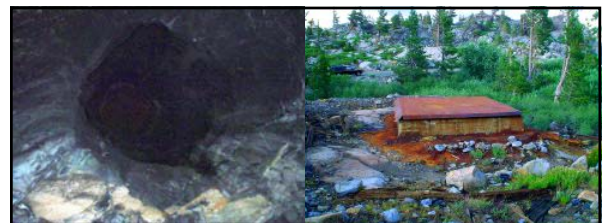
Left: the vertical central shaft of the CPRR's Summit Tunnel (a.k.a. Tunnel No. 6) at Donner Summit which allowed drilling and excavation to be carried out on four faces simultaneously. The 125-foot deep shaft provided four working faces, speeding-up progress significantly. With much difficulty, the steam engine of an old locomotive was brought up the wagon-road and used as a winch driver to help remove loosened rock from the four working faces. A winter camp was established. However, the trail down from the camp grew so dangerous (due to snow-slides) that all work was stopped. The slides carried away camps and crews. In the spring of 1867, the frozen corpses of laborers were revealed as the snow level dropped; still upright, their tools frozen in their hands. The Summit Tunnel was a year in the making, complete by August 1867.
