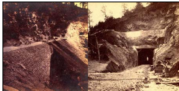
Left: caption: "Horse Ravine Wall and Grizzly Hill Tunnel" Right: caption: "Grizzly Hill Tunnel from the North"
