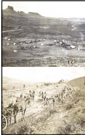
Top: an overview of one of the main UPRR camps as the line pushed west. The presence of crude wood buildings in addition to tents suggests more infrastructure is being sent to this point, which indicates a longer stay for a larger number of residents. Bottom: this photograph depicts a classic scene along the construction of the transcontinental RR. Workers lay track while horse-drawn carriages bring supplies alongside.
