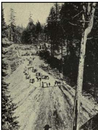
Left: caption: "Building Through the Forest - C.P.R.R., Sierra Nevada Mountains, 1864." Hills and/or ridges in front of the road bed would have to have a flat-bottomed, "V"-shaped cut to get the tracks past (the nature of the material determined the slope and how much material would have to be removed). Ideally, these cuts would be matched with valley fills that could use the "spoil" to bring the road-bed up to grade (a.k.a. "cut & fill" construction). At the time, there was no heavy equipment that could be used to make the cuts and/or haul it away to make the fills. The only options were to dig it out manually by pick and shovel, haul the spoil by wheelbarrow and/or horse/mule cart or blast it loose. To blast a V-shaped cut, several holes were drilled (up to 20-feet deep), filled with black powder and the material blasted away. Unfortunately, the explosive technique often blew most of the potential fill material down the hillside, making it unusable as fill.
