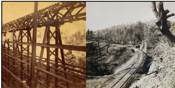
Left: caption: "Trestle Bridge, Clipper Ravine, near view" Right: caption: "View above Clipper Gap, Placer County"
