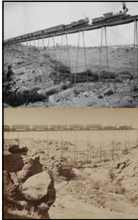
Left T&B: this later, steel version of the Dale Creek Bridge was abandoned after the UPRR line was moved a few miles south in 1899
