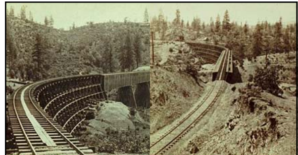
Left: caption: "Long Ravine Bridge – 120 feet high, 878 feet long" Right: caption: "Long Ravine Bridge, overhead view"
