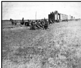
"...Thirty seconds to each pair of rails; two rail lengths to the minute, three blows to each spike, ten spikes to a rail, 400 rails and 4,000 spikes and 12,000 blows to a mile. To every mile some 2,500 ties - say 2,400 at the outset, 2,650 on the grades - at $2.50 each, delivered. The roadbed is ever calling for more and more..."
