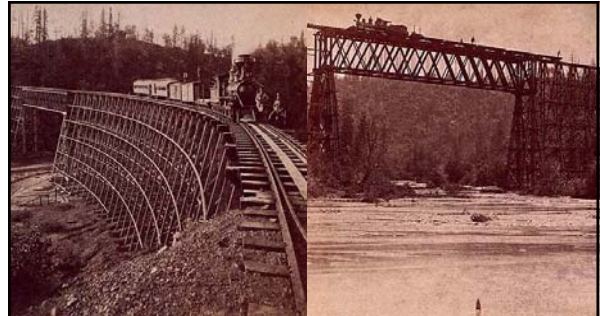
Left & Right: caption: "Railroad Trestle Work crossing Bear River, Cal." 664
