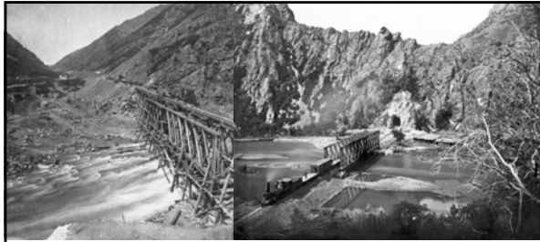
Left: UPRR crews construct a trestle over the Weber River, Utah during the winter of 1869. Devil's Gate in Weber Canyon was one of the final obstacles crews overcame before reaching Promontory Summit. Right: the UPRR's last geographic obstacle before reaching Promontory Summit came in the form of a series of tunnels through hard rock in Weber Canyon. This image shows a construction train crossing a trestle bridge after exiting the eastern portal of Tunnel No. 3.
