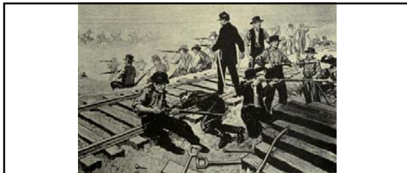
"Every mile had to be run within range of the musket. In making the surveys numbers of our men, some of them the ablest and most promising, were killed; and during the construction our stock was run off by the hundred, I might say by the thousand; our cars and stations and ranches burned. Graders and track-layers, tie-men and station-builders, had to sleep under guard, and have gone to their work with their picks and shovels and their mechanical tools in one hand and the rifle in the other, and they often had to drop one and use the other." Grenville Dodge, UPRR Chief Engineer Above: caption: "Defending the Rails, 1867" 563
