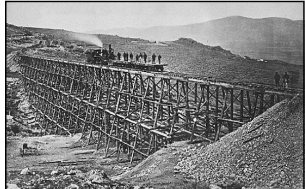
Above: caption: "Trestle Work – Promontory Point, Salt Lake Valley, Utah" 306
