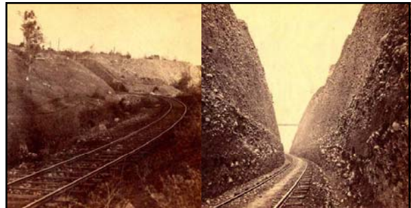
Left: caption: "Approaching Bloomer Cut from the West" Right: caption: "Bloomer Cut, looking East – 800 feet long and 65 feet high"
