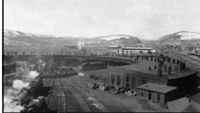
Bottom: view of the UPRR roundhouse in Rawlins Wyoming (showing locomotives, trains, turntable & shops)
