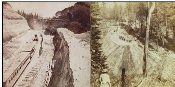
Left: caption: "Hog's Back Cut. 60 feet deep. 2 miles above Alta." Right: caption: "Grading the Central Pacific Railroad – Sailor's Spur and Fill. 12 miles above Alta, Placer County."
