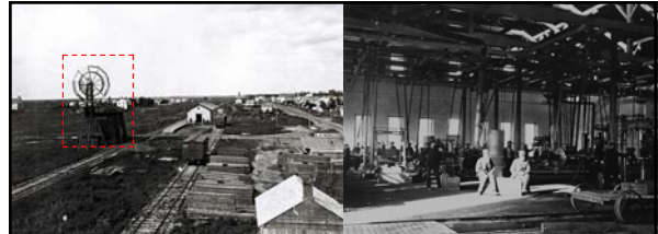
Above: inside Laramie's UPRR machine shops Left T&B: a windmill at Laramie drew water for steam locomotives. Roundhouse and machine shops at back right.
