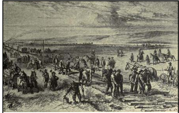
Above: caption: "Westward Across the Plains, 1866.' An excellent sketch of the Union Pacific R.R. in construction through Nebraska." 488
