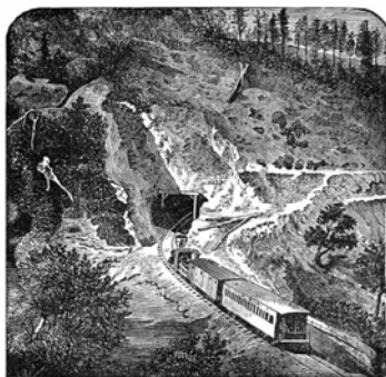
No. 116—WEST PORTAL, TUNNEL NO. 1, C. P. R. R.
