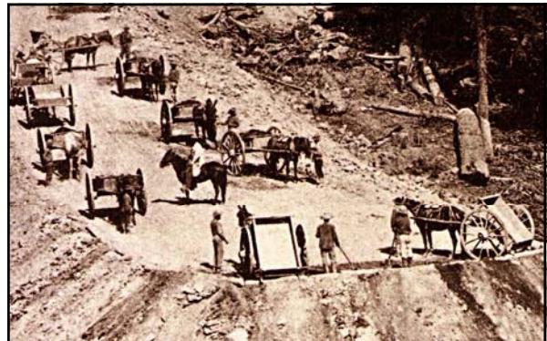
Above: caption: "Bank and Cut at Sailor's Spur. 80 miles from Sacramento."
