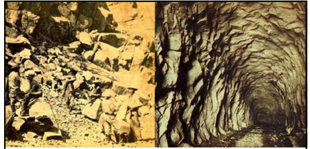
Left: caption: "Laborers and Rocks, near opening of Summit Tunnel"
