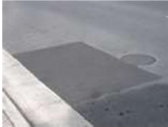
Special Pavement Patching (Steve Muench; hawaiiiasphalt.org)
