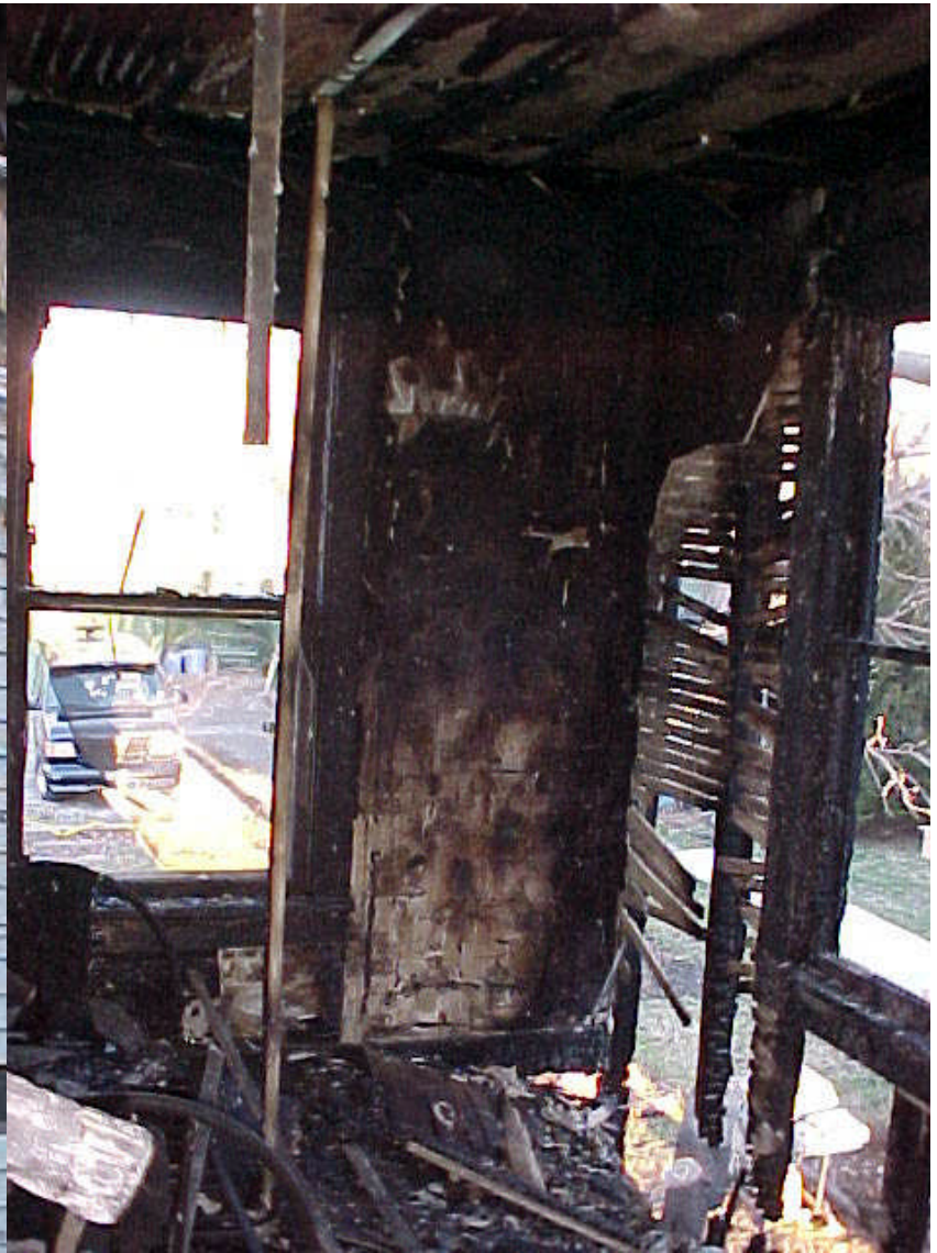
Left: caption: “Results of fire extension from kitchen window up to rear bedroom”
