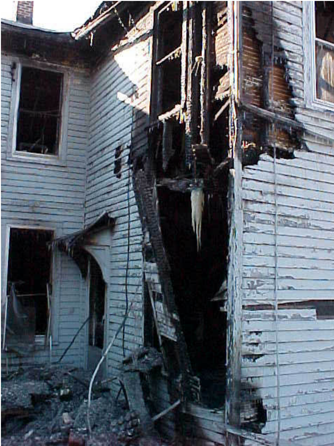
Left: caption: “Results of fire extension from kitchen window up to rear bedroom”
