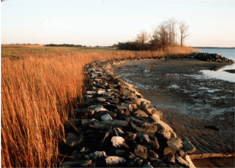
a. Stone sill with marsh planting on Chester River, Kent County, MD
