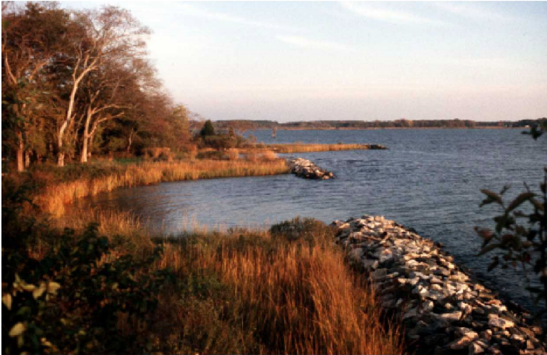
c. Breakwater and sill project after 5 years
