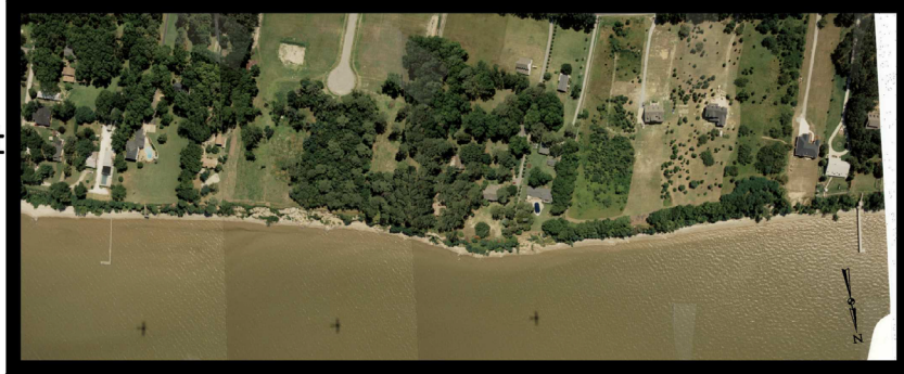
VanDyke Project Pre-Construction 1994
