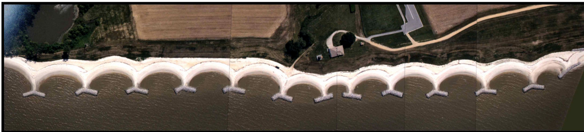
Luter Project One year after construction, May 1999 Approximate photo scale 1 inch=200 ft
