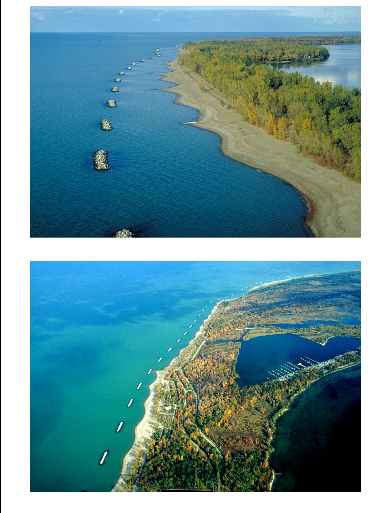
Figure V-3-19. Breakwater construction and salients; two views of Presque Isle, Pennsylvania (from Mohr 1994)
