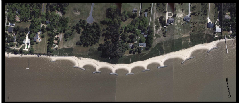
VanDyke Project Two Years After Construction 1999
