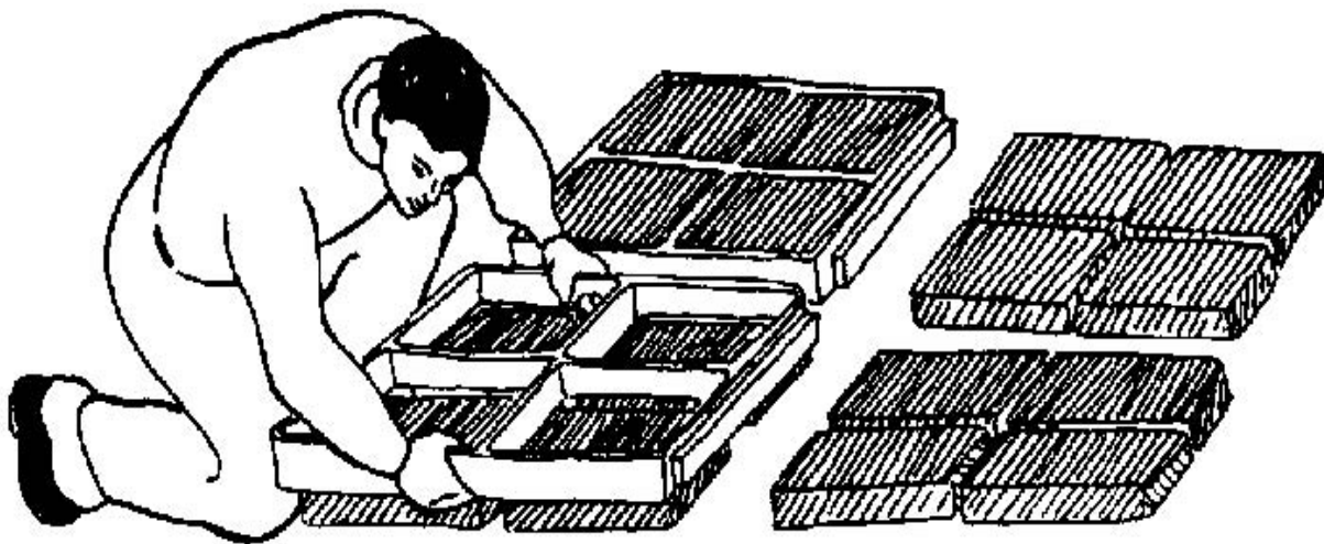
Figure 41. Lifting the forms from freshly made blocks.
