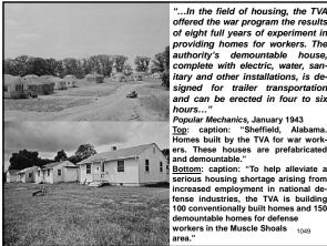
offered the war program the results of eight full years of experiment in providing homes for workers. The , authority's demountable house, complete with electric, water, san itary and other installations, is designed for trailer transportation and can be erected in four to six
