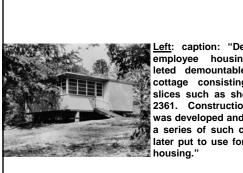
\_eft: caption: "Demountable employee housing. Completed demountable vacation cottage consisting of four slices such as shown on K-2361. Construction method was developed and proved on a series of such cabins, and later put to use for employee
