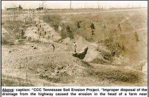
drainage from the highway caused the erosion in the head of a farm nea Demoray. Plank check dams were built in the main gully, with a masonry soil saving dam constructed at a point where it would catch a considerable <sup>319</sup> amount of sitt. The further treatment of this area will be to plant locust and pine."
