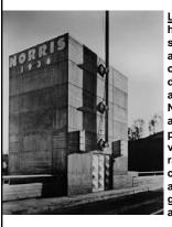
Left: caption: "Elevator penthouse atop dam which also serves as flagpole base. Elevator serves various levels of operating machinery inside dam. Top of dam is developed as roadway with sidewalks Note handrail projecting toward sidewalk and toe space in parapet to make enjoyment of view more comfortable. Handrail brackets are hollow and contain lights which illuminate the roadway but avoid glare by the use of reflectors and directional lenses." 178
