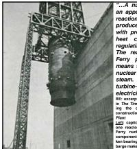
"...A nuclear reactor is simply an apparatus in which a chain reaction, the splitting of atoms to produce heat, can take place with precision and safety. The heat can be controlled by regulating the nuclear reaction. The reactors for the brown's Ferry plant use water as a means to absorb heat from the nuclear reaction to produce steam. The steam turns the turbine-generators that generate electricitv..."
