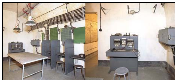
Left: caption: "Telephone booths in the artillery commanders post for communicating with the blocks" Right: caption: "Switchboard in the artillery commanders post"
