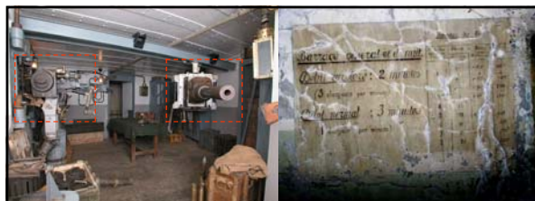
Left: caption: "One of the firing rooms of interval casemate Grand Lot. Visible on the left side is one of the embrasures with a JM Reibel. The 47mm AT gun can be seen mounted on the rail on the right."
