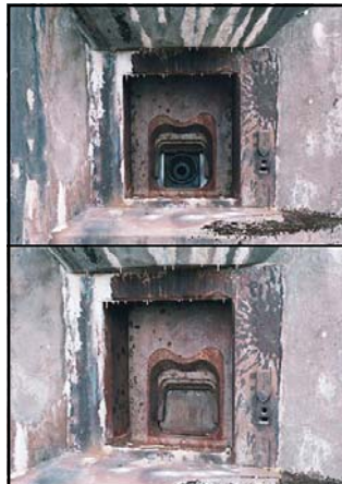
Left: caption: "The vertical sliding armored shutter of the embrasure. Note the shell splash just above the optics opening on the embrasure." 449
