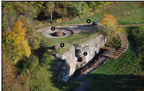
Above: caption: "A picturesque view of Artillery Block 9 of GO Hackenberg. 1) embrasure for one 135mm model 1932 howitzer 2) 135mm gun turret 3 & 4) GFM cupolas" 447
