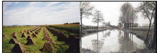
Tank traps were also built for miles along the Siegfried Line and were known as "Dragon's Teeth" or "Pimples" (in German: Hocker = "humps") because of their shape. These blocks of reinforced concrete stand in several rows on a single foundation. There were two typical sorts of barrier; Type 1938 with four teeth (getting higher toward the back) and Type 1939 with five such teeth (left). Many other irregular lines of teeth were also built. Another design of tank obstacle was made by welding together several bars of steel in such a way that any tank rolling over it would be penetrated in its weak bottom armor. If the lay-of-the-land allowed it, water-filled ditches were dug instead of tank traps. An example of this kind of defense are those north of Aachen near Geilenkirchen (right).
