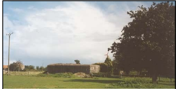
The Geldern Emplacement lengthened the Siegfried Line northwards as far as Kleve on the Rhine River and was built after the start of WWII. The Siegfried Line originally ended in the north near Bruggen (in the Vierseen District ). The primary constructions were unarmed dugouts which were extremely strongly built out of concrete. For camouflage, they were often built near farms.
