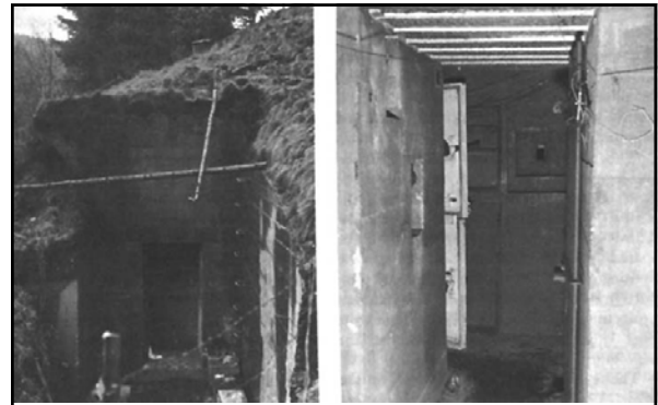
Above L&R: caption: "Typical Pillbox. Exterior (left), showing door with firing embrasure. Interior of firing embrasure (right)."
