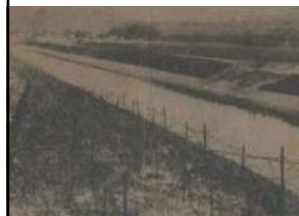
Left: caption: "A front view of the 'Limes' or Siegfried Line of Germany, which has hurriedly been completed during the last year, reveals a formidable barrier of barbed wire. The barbs are said to be scientifically intertwined to give the most trouble to an approaching enemy. Notice, too, the moat, or canal, which extends in front of the fortification to form an added barrier."
