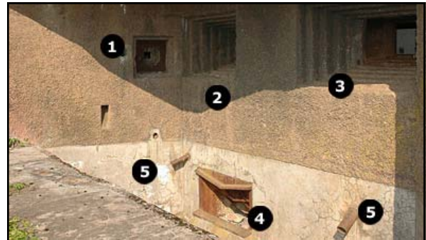
Above: caption: "1) Close-in defense (7.5mm) 2) Twin machine-gun position 3) Twin machine-gun position + anti-tank gun 4) 50mm mortar 5) Spent cartridge exit tubes" 362
