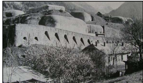
In the Alps, not all the casemates had weak walls since several artillery casemates actually faced the enemy line of advance. These casemates not only had thicker walls, but also more armor protection. This was done because in many positions the engineers could not justify the employment of an expensive artillery turret which would have a limited field-of-fire.
