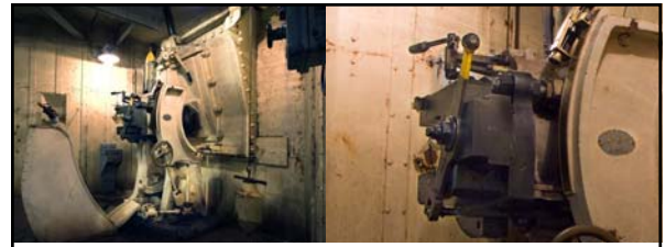
Left: caption: "Underneath the lamp, mounted against the wall, is a device which could 'merge' the shell and the cartridge case. In the bottom right corner hangs a weight, attached to a steel wire, to close the armored slide on the outside. In the top right corner a silhouette of a remote fire-directing device, while a grenade-launcher is visible on the left, just above the voluminous spent case bin." Right: caption: "A detail of the rear of the gun" 448
