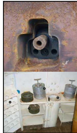
Top: caption: "The business end of one of the AM units. The barrel of the 25mm anti-tank gun can be seen, as well as the two mini-em-brasures for the MAC 31 machine-guns. The hole in the middle is for the optics device of the gunner."
