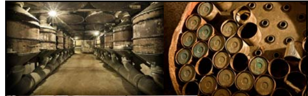
Top Left: caption: "Decontamination (filter chamber) room in GO ouvrage Galgenberg"
