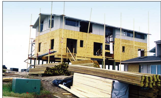
Figure 2. Vertical addition to a home damaged by Hurricane Fran. Preexisting 1-story home became the second story of a home elevated to meet new foundation and floor elevation requirements.
