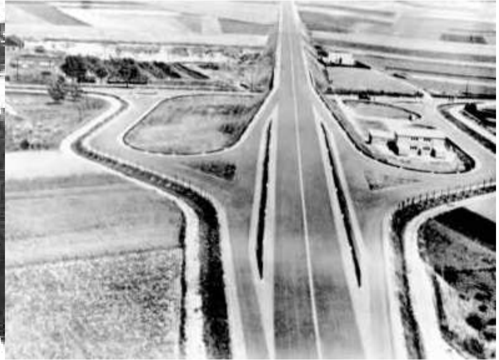
Above: caption: “The first European motorway junction (1932)”
