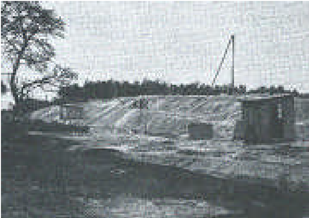
Fig. 2. Swamp blasting; sand fill before explosion
