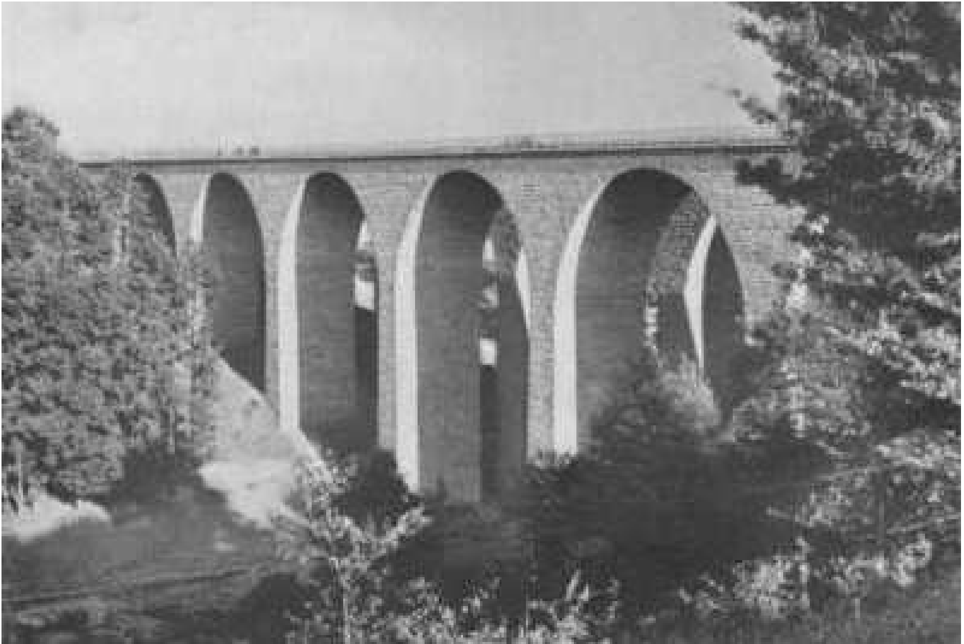
Above: caption: “The Waschmuhltal Bridge for Autobahn A6 at Kaiserslautern was built to a design by Fritz Todt and Paul Bonatz”
