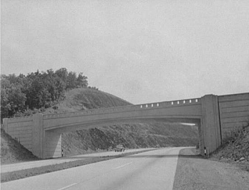
Above & Left: typical PT overpasses
