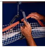
3. Place cable in mesh. Secure with steel retaining strap. (The removable retaining strap allows for future cables.)
