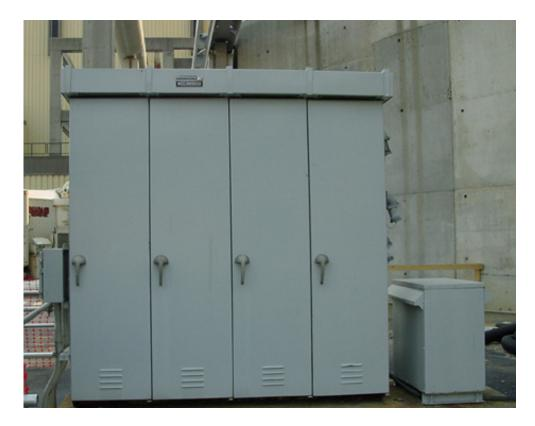
Motor Control Centers are located throughout the power plant and are placed near groups of loads for convenience. Outdoor MCCs are located in an additional enclosure for weather protection. A door opens to reveal each vertical section as shown in the photo above.
