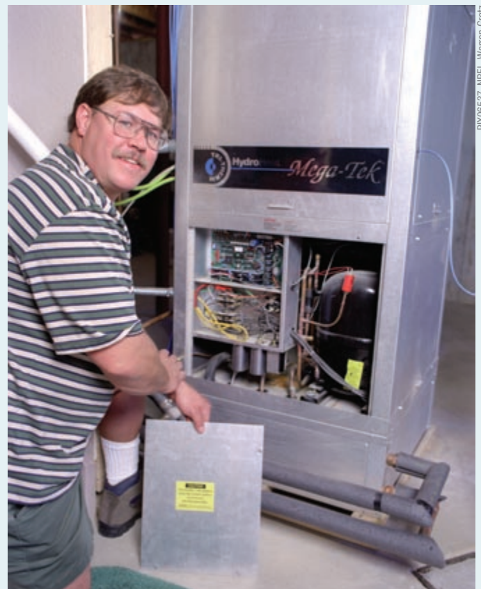
Residential application of a geothermal heat pump in Colorado.
