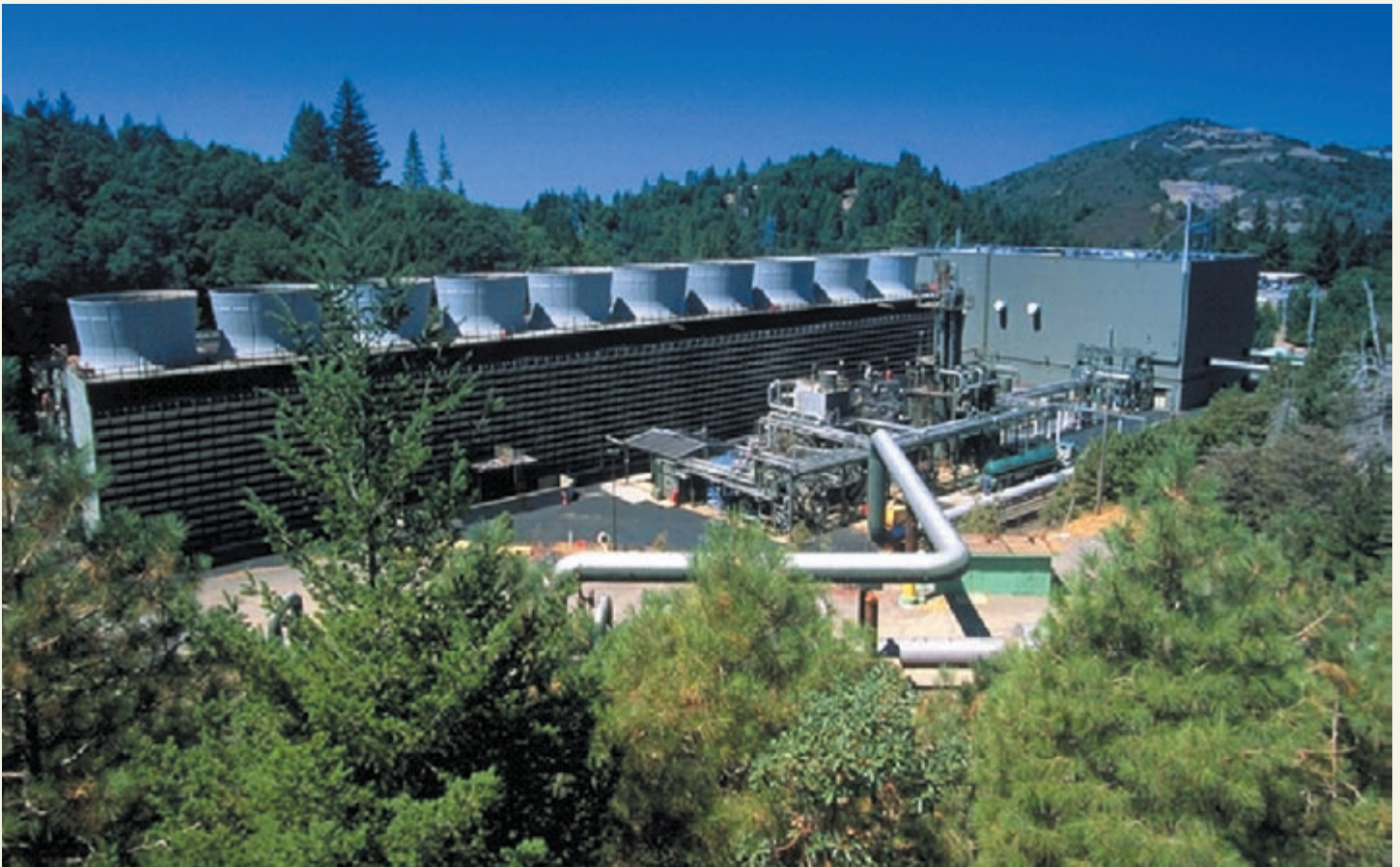
Big Geysers, Unit 13, a 75-MW geothermal power plant located in northern California. Credit - Calpine Corp.
