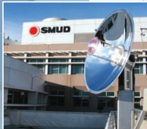
Oak Ridge National Laboratory installed a hybrid solar lighting system at Sacramento Municipal Utility District's Customer Service Center (left). Sunlight collected by such a system is routed through optical fibers to provide interior lighting (right).
