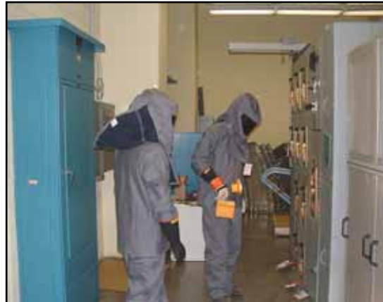
Figure 8. – Example arc flash protective gear. Level of protection required is dependant on available arc flash energy.
