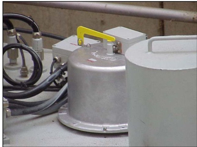
Figure 10.— Pressure Relief Device.
