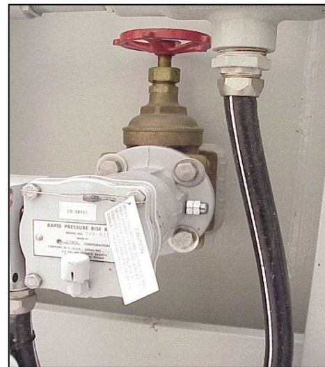
Figure 12.—Sudden Pressure Relay.
