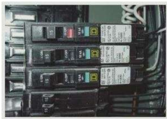
Photo 2. AFCI, single circuit breaker type
