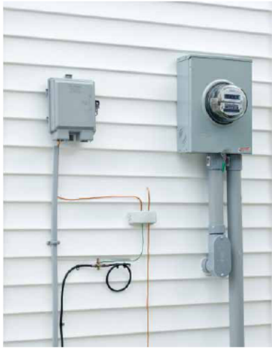
ERITECH Intersystem Bonding Termination - Typical installation bonding the electrical system to the telephone and CATV systems.
