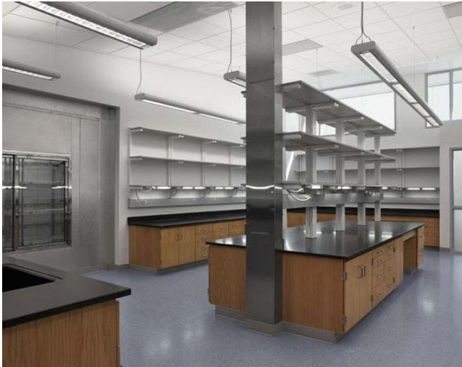
Figure 7. Under-cabinet task lighting in a USDA laboratory. Source: HOK.
