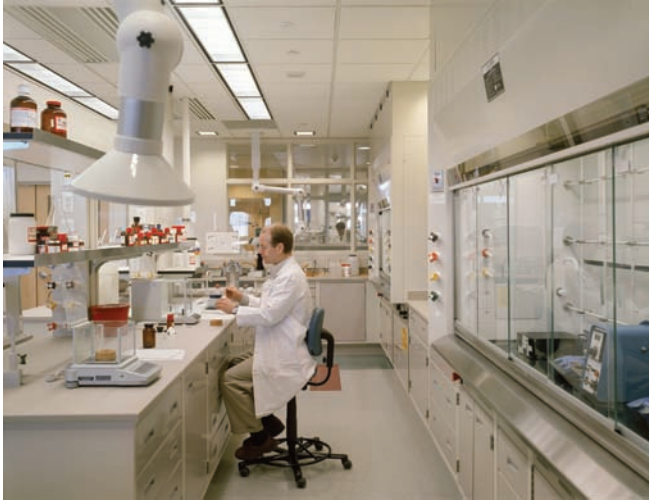
Figure 10: Balance of surface brightness in this lab is achieved with energy-efficient recessed lab lighting using T8 technology and compact fluorescent down lights with 4100-K lamp color. Photo courtesy of Pivotal Lighting Design/Affiliated Engineers.
