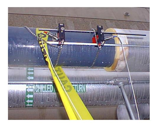
Figure 6: Ultrasonic 'strap-on' temporary flow meters
