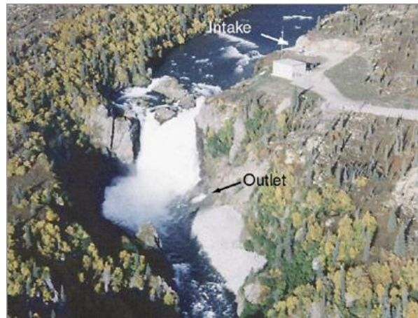
The Tazimina Hydropower Plant (DOE Photo)
