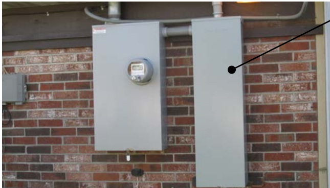
Service disconnect and branch circuit breakers (panelboard)
