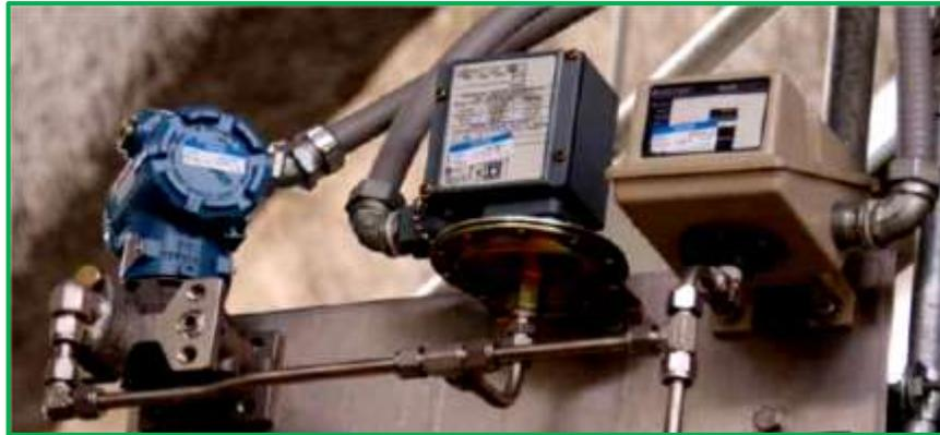
One of the settings on this switch is the “*deadband*” or “*differential pressure*” setting to determine the amount of pressure change required to re-set the switch to its normal state after it has tripped. For example, a high-pressure switch with a trip point of 67 PSI increasing, that re-sets back to its normal state at a pressure of 63 PSI decreasing, then this pressure switch has a “*deadband*” or “*differential*” pressure setting of 4 PSI (67 PSI – 63 PSI = 4 PSI).
