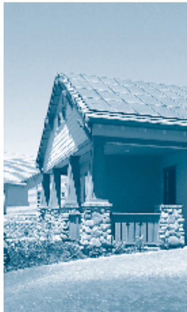
Photovoltaic System, Centex Homes, Livermore, CA
