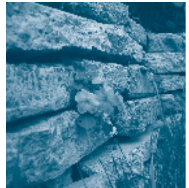
Recycled concrete wall (urbanite).
