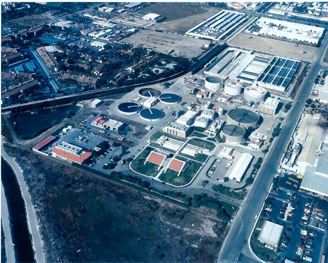
Figure 1: Aerial View of Oxnard Wastewater Treatment Plant (Photo provided courtesy of Oxnard WWTP)
