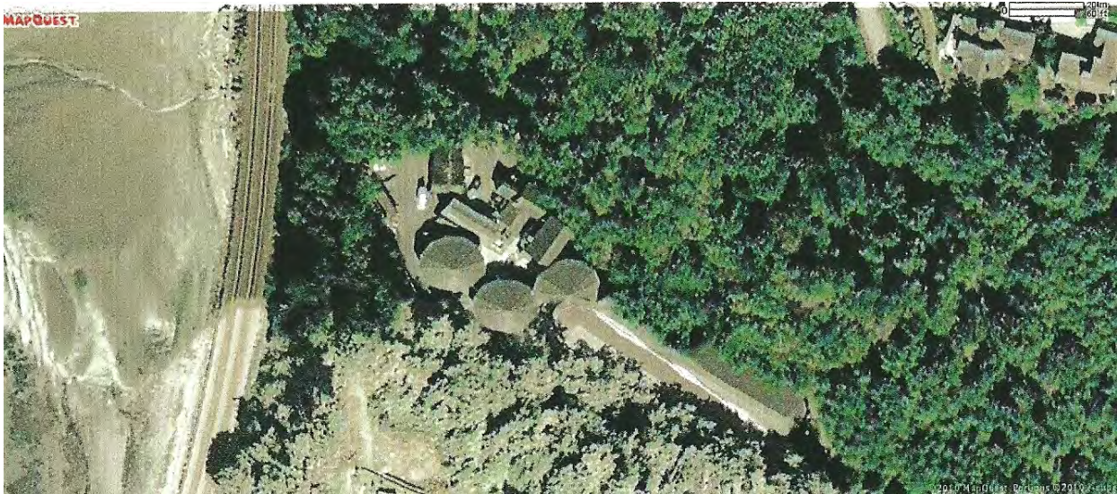
Figure 1: Aerial View of Big Gulch WWTP
