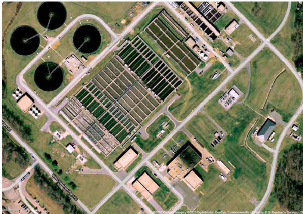
Figure 1: Washington Suburban Sanitary Commission Western Branch WWTP
