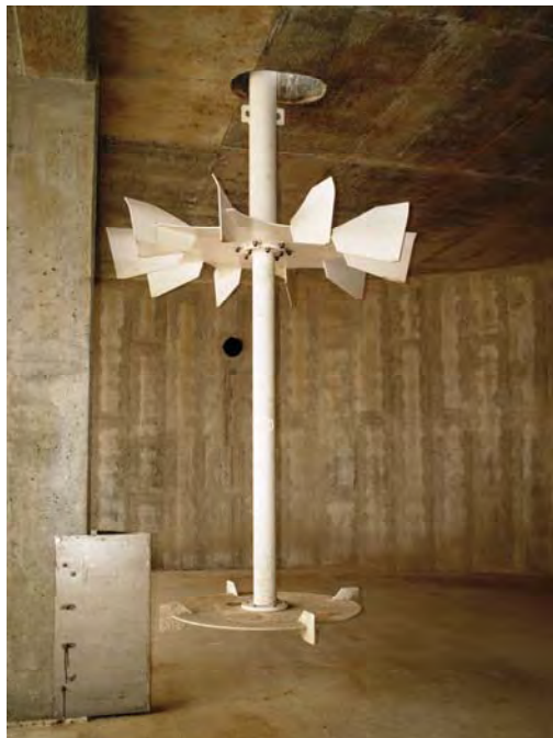
Figure 4-1. Eimco Water Technologies Carousel ® System Excell ® Aerator II Source: Eimco Water Technologies. Used with permission.
