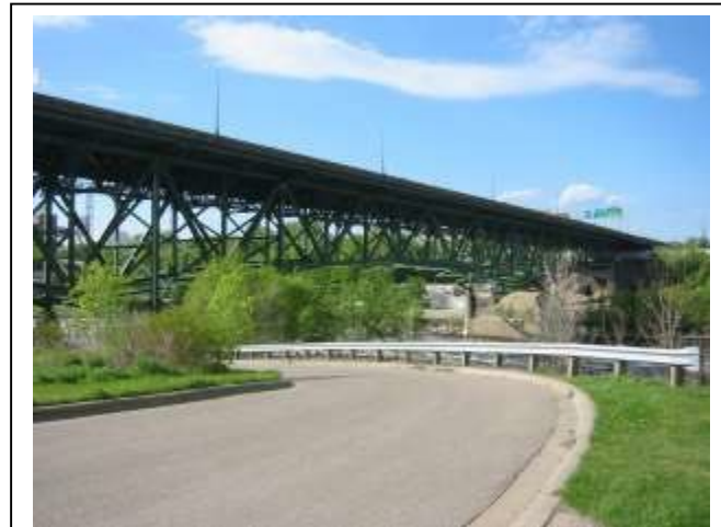
I-35W Highway Bridge before collapse
