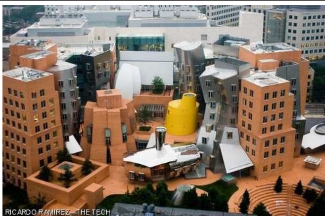
RICARDO RAMIREZ—THE TECH The Ray and Maria Stata Center at MIT defies some natural laws governing construction. Photo: The Tech
