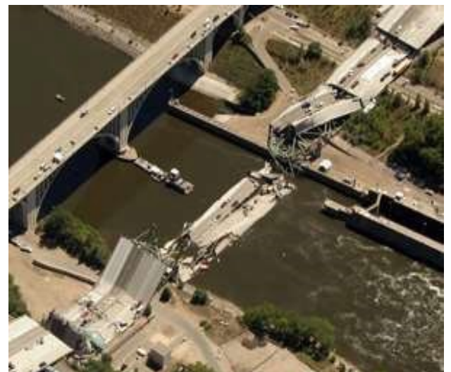
I-35W Highway Bridge after collapse Photo: NTSB
