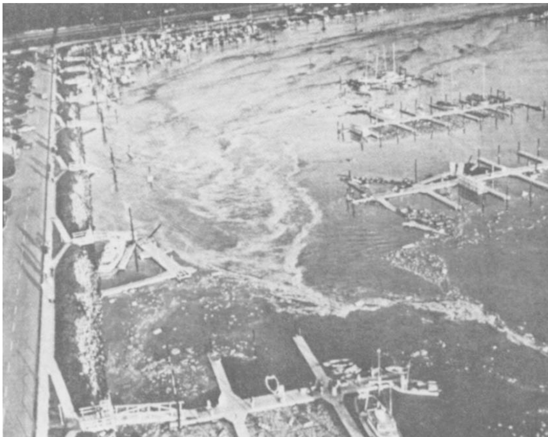
Figure 3-2. River flood damage at Ventura Marina, California.
