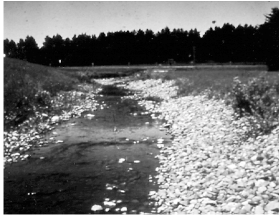
Figure 29. Riprap channel lining.
