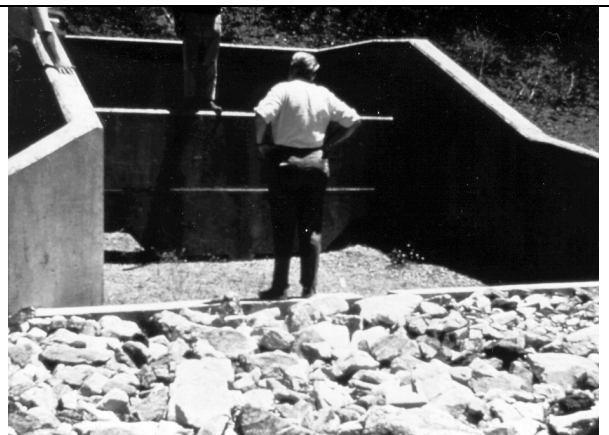
Figure 51b. Baffle-wall energy dissipator - USBR Type VI.
