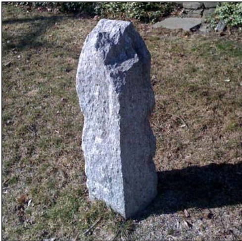
Figure 16. Ancient granite corner, approx. 9" x 12" x 5'.
