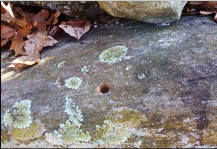
Figure 23. Old drill hole at a corner, widened during a recent survey.
