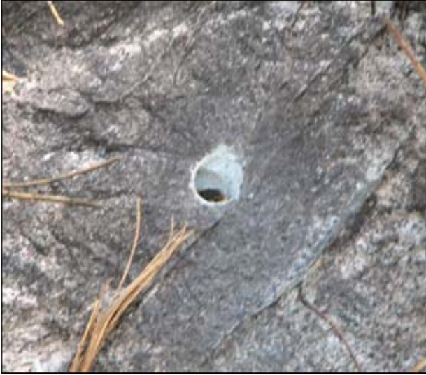
Figure 10. A new drill hole in a stonewall.
