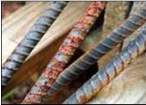
Figure 19. Typical rebar stored outside for use as corners.
