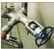
Class 2500 hermetically-sealed Y-pattern bellows sealed valves.
