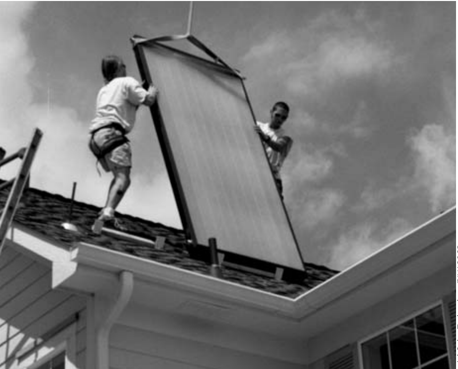
Specialists can safely and efficiently install solar thermal systems
