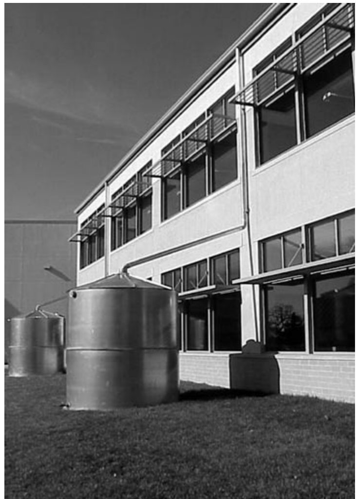
This exterior view of the Nidus Center for Scientific Enterprise in St. Louis, Missouri, shows the cisterns that store rainwater used to irrigate the grounds of this research facility.
