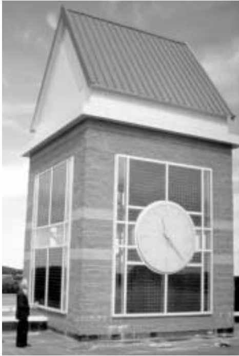
Pilkington Solar International's project leader, John Goldsmith, is shown with the integrated curtain wall on the south and west faces of the clock tower.
