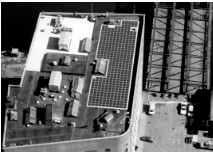
Co-funded by the DOE FEMP Renewable Energy Program, this BIPV application illustrates how the technology can be introduced into complex roof spaces.
