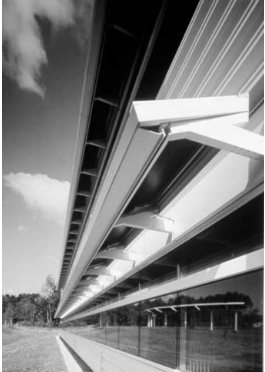
Close-up view of photovoltaic sunshade
