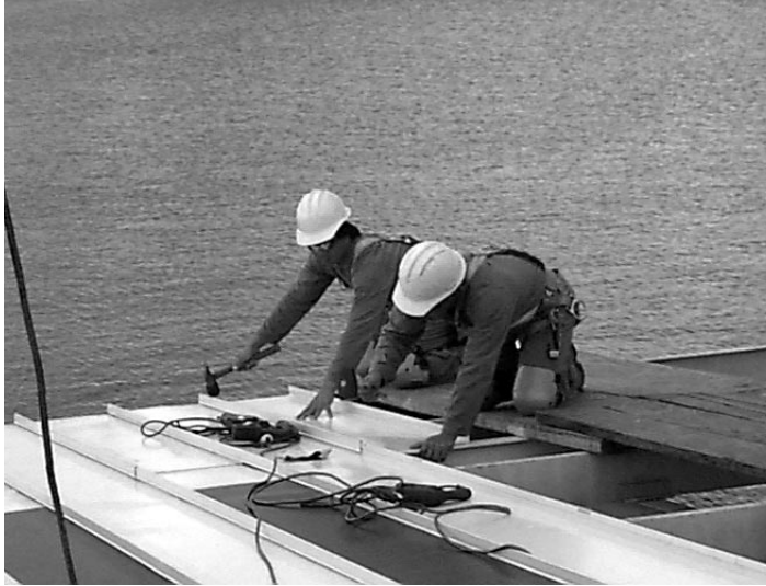
Workers install short lapped roofing pans at BIPV module sections.
