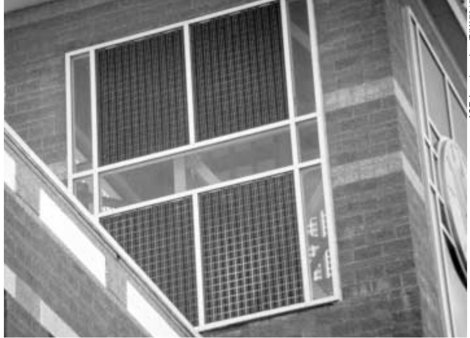
East view of the clock tower shows BIPV installation.
