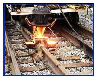
Aluminothermic, Exothermic or Thermite Welding is described in the AWS Welding Handbook, Section 2. It is a process that employs a reaction between iron oxide and aluminum producing a red hot iron slag, which is the filler material, through a **chemical reaction called exothermic** or aluminothermic.
