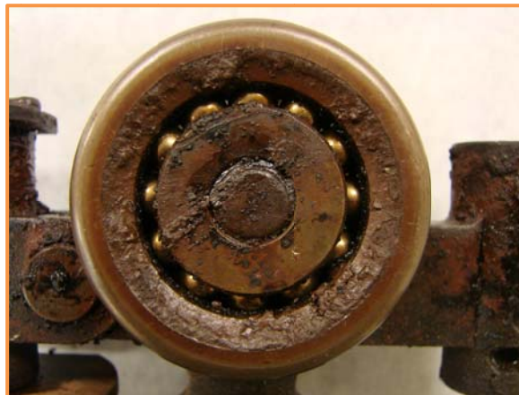
Lubrication grease compromised by water ingress
