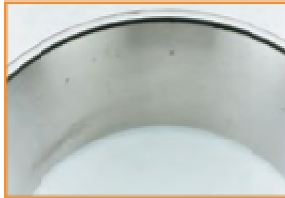
Roller spaced nicking: raised metal on race from contact with roller edges
