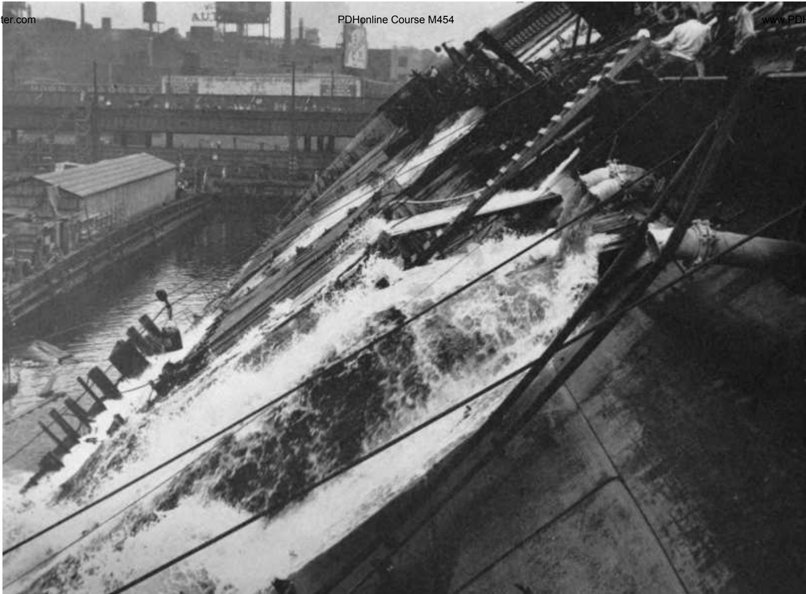
Ship at 45-degree inclination (during pumping-out operation)
