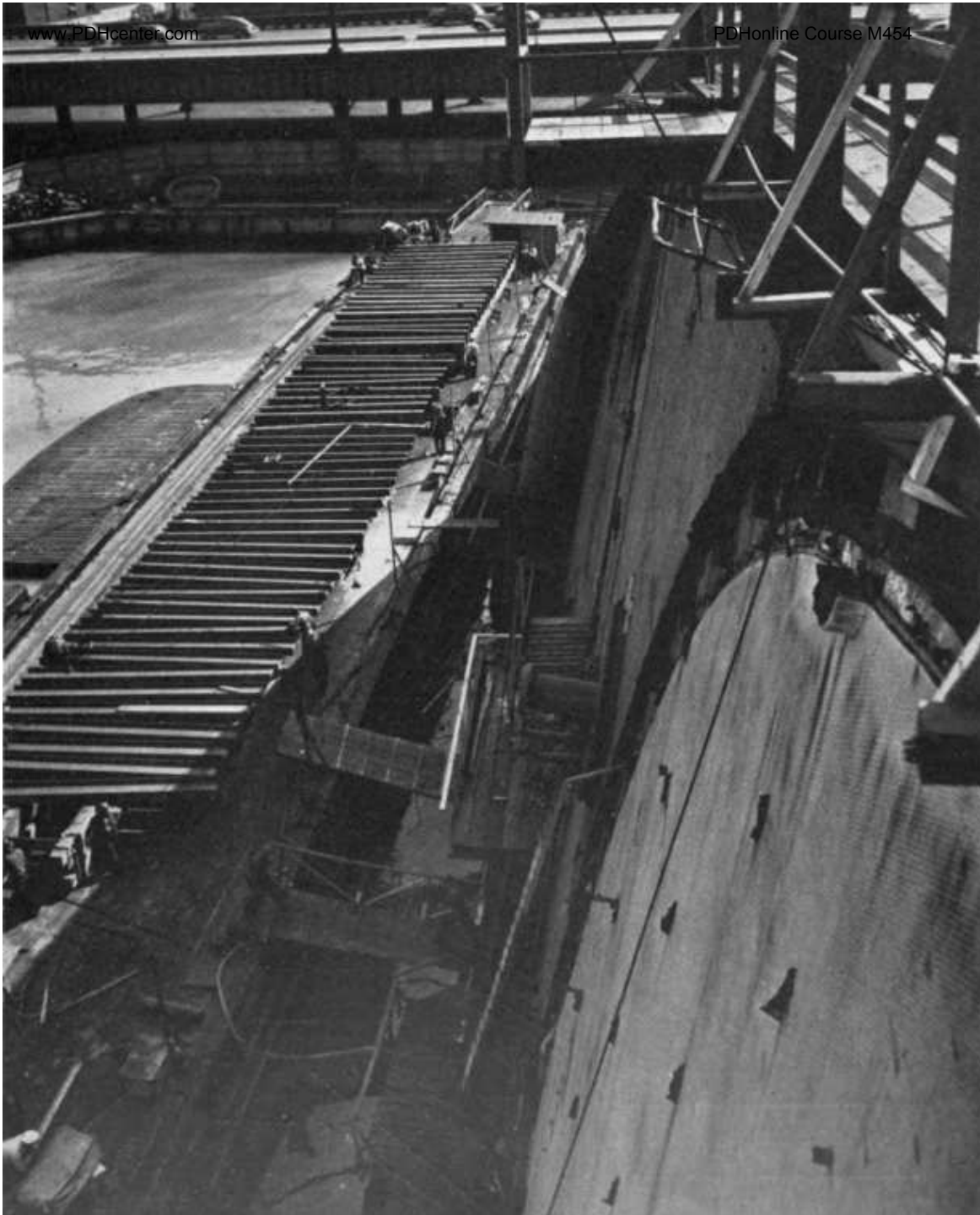
Left: Barge aside the Promenade Deck where the large cargo port patch was constructed
