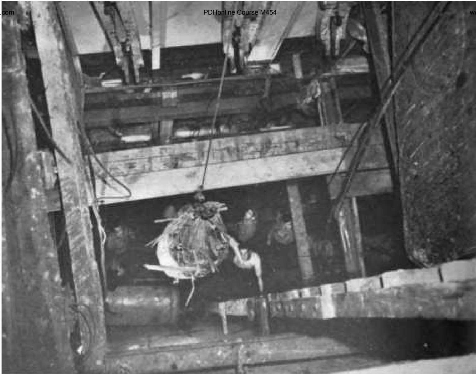
Hoisting rubble through open cargo door
