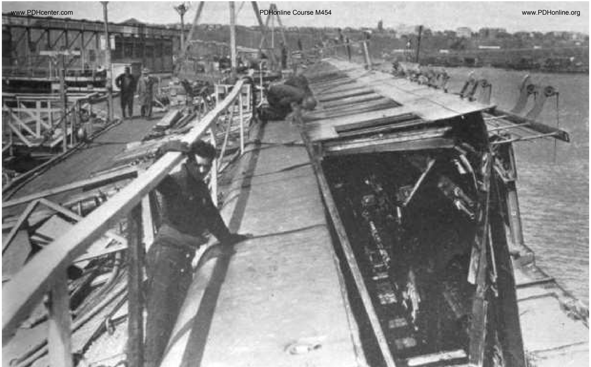
Removing structure above Promenade Deck
