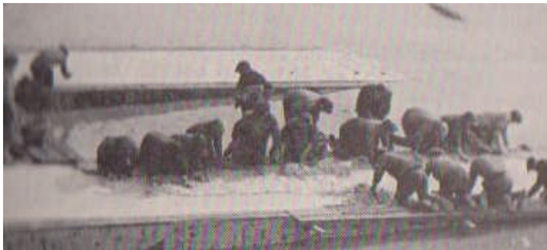
Left: greasing the “Standing Ways”
