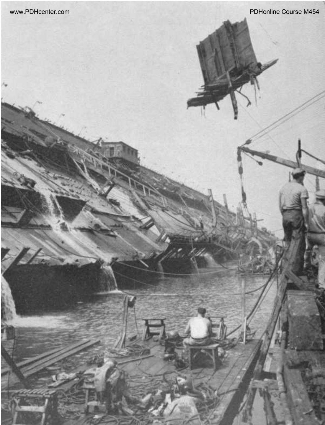
Removing remaining portion of superstructure
