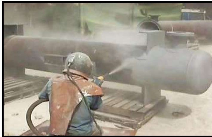
SSPC-SP5/NACE 1: White Metal Blast Cleaning
