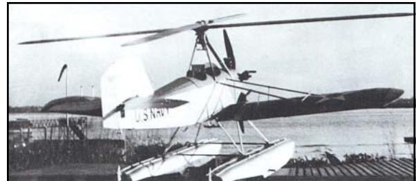
The U.S. Navy's XOZ-1 autogiro was a Consolidated N2Y-1 tandem-seat biplane trainer rebuilt in the mid-1930s as an Autogiro. These planes were used as familiarization trainers for the Navy "skyhook" pilots who flew fighters from the large Navy airships USS Akron and USS Macon . The XOZ-1 was modified to an Autogiro configuration by the Pennsylvania Aircraft Syndicate , with a four-bladed Autogiro rotor held aloft over the forward cockpit by four steel struts, replacing the upper wing. The lower wing was retained, supports added and the wheeled undercarriage was replaced by twin floats. The two-bladed wooden airscrew was retained as were the two open, tandem cockpits. The aircraft was tested by 370 the National Advisory Committee for Aeronautics (NACA) .
